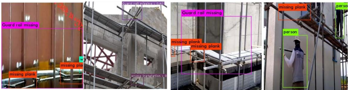
Figure 3: Example of scaffold components for Tools Inspection Before Work
