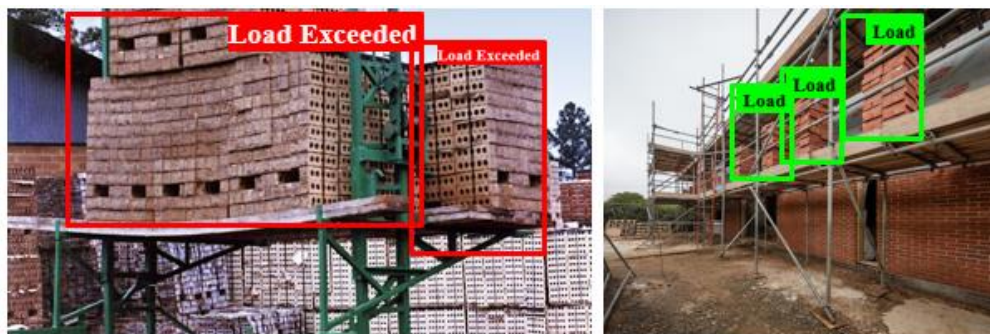
Figure 7: Example of loaded Scaffolds for Monitoring During the Whole Work
