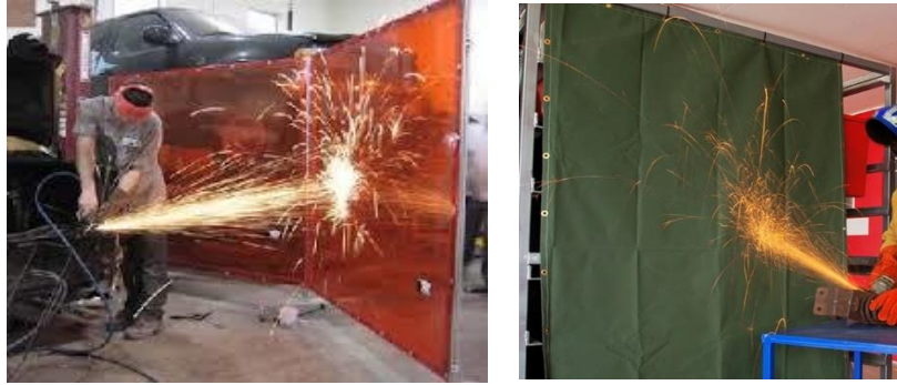
Figure 2: Example of Welding Activity for Safety Equipment Installation Before Work
