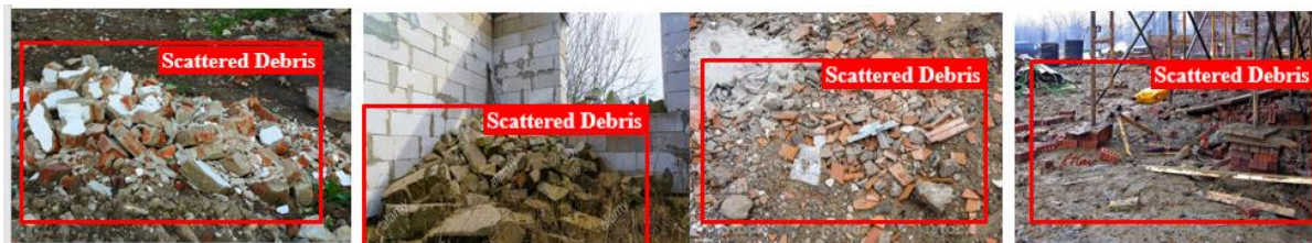
Figure 4: Example of Broken or Scattered Masonry for Monitoring with Intervals
