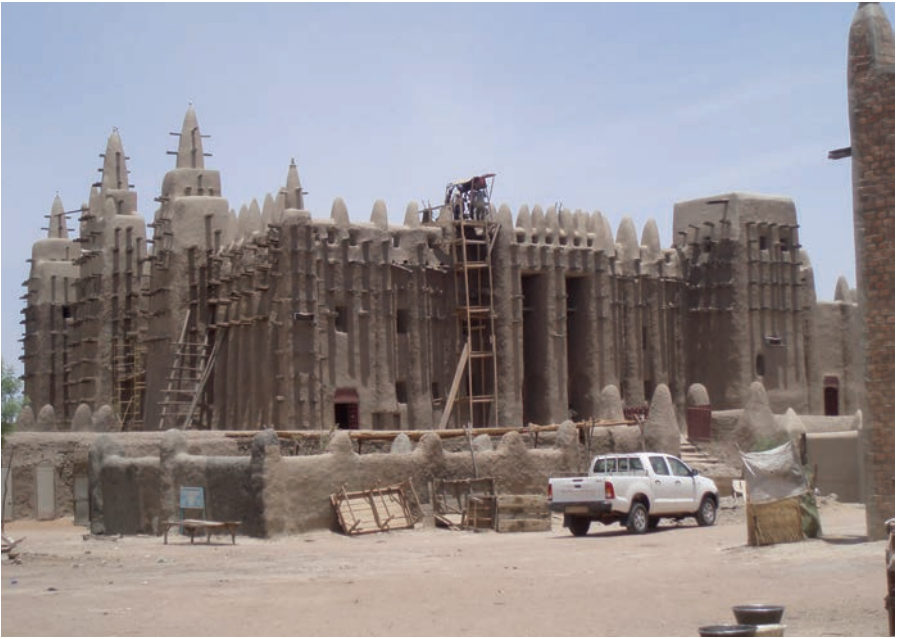
Plate 15 An early stage in the AKTC restoration works JOSEPH BRUNET-JAILLY
