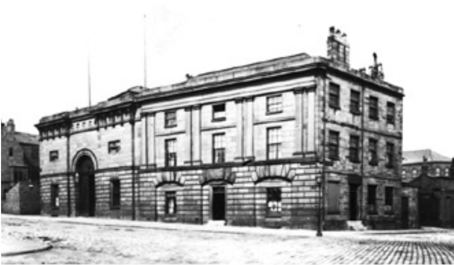
37. Riding School, 1846–7 (subsequently altered, left) and Zetland Hotel, 1846–7 (right), Ramsden Street (now Queensgate), Huddersfield, both by William Wallen.
