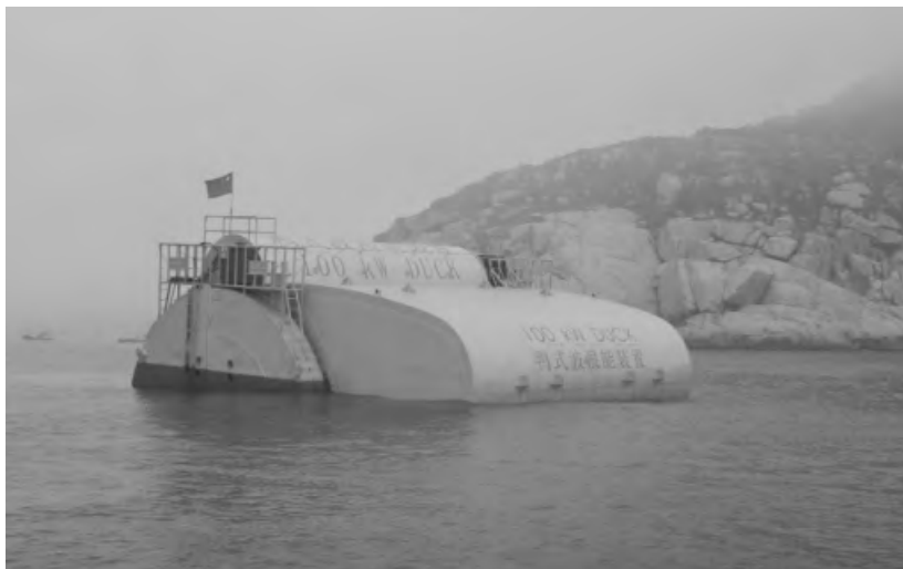
Figure 1.16: Pitching Duck type WEC constructed by the Guangzhou Institute of Energy Conversion, at the Chinese Academy of Sciences, (image courtesy of Guangzhou Institute of Energy Conversion).
