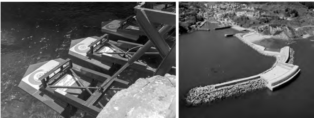
Figure 9.2: (a) An Eco Wave Power array, installed at a former World War II Ammunition Jetty in Gibraltar and providing 100 kW to the electric grid. (b) A birds-eye view of the Mutriku wave power plant, consisting of 16 oscillating water column chambers installed at a breakwater structure [108]. Pictures republished under the Creative Commons CC-BY-SA-4.0 license.
