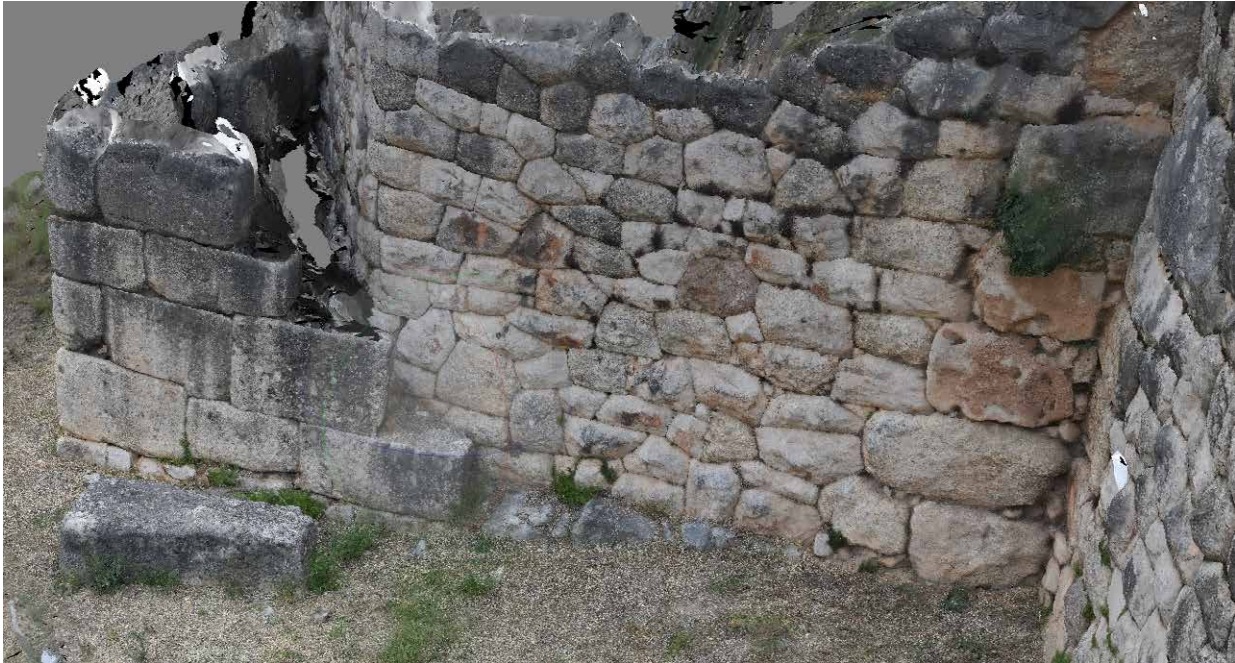
Figure 3.6 View on the backside of the bastion at the Lion Gate, Mycenae (textured 3D model by author). The cut blocks on the left form a separate façade around the wall (note that this section of wall is not cyclopean). It also shows the somewhat irregular shape and size of these conglomerate blocks, as mentioned by Küpper, which makes that he does not consider them as true ashlar.
