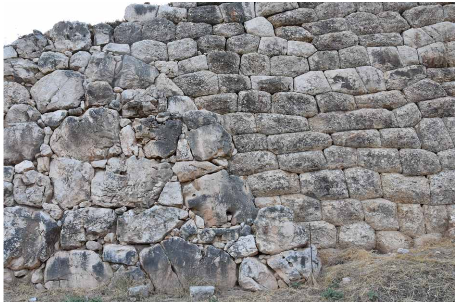
Figure 3.2 Top: Cyclopean-style wall. Part of the fortification at Mycenae. Bottom: difference between the cyclopean-style section (left) and the later Hellenistic polygonal-style section (right). Note the well-fitting blocks in the Hellenistic section. Each block had to be cut specifically to fit. Also, note that many blocks on the left are quite a bit larger than those on the right (photographs by author).
