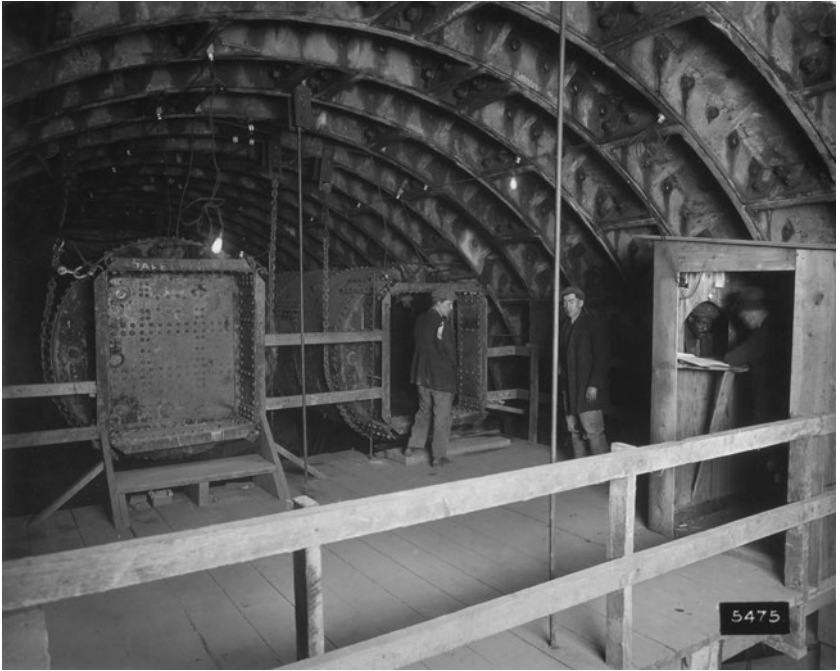
Man lock, south tunnel, New York
