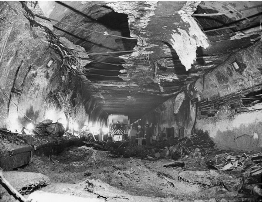
Top: burned truck in south tunnel, May 13, 1949; bottom: south tunnel, May 14, 1949
