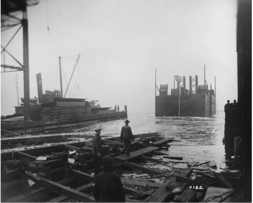
Launching of New Jersey north river caisson, Staten Island
