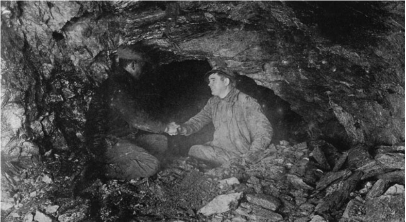
Top, left: men tightening bolts; top, right: grout nose and nipple in plate; bottom: holing through
