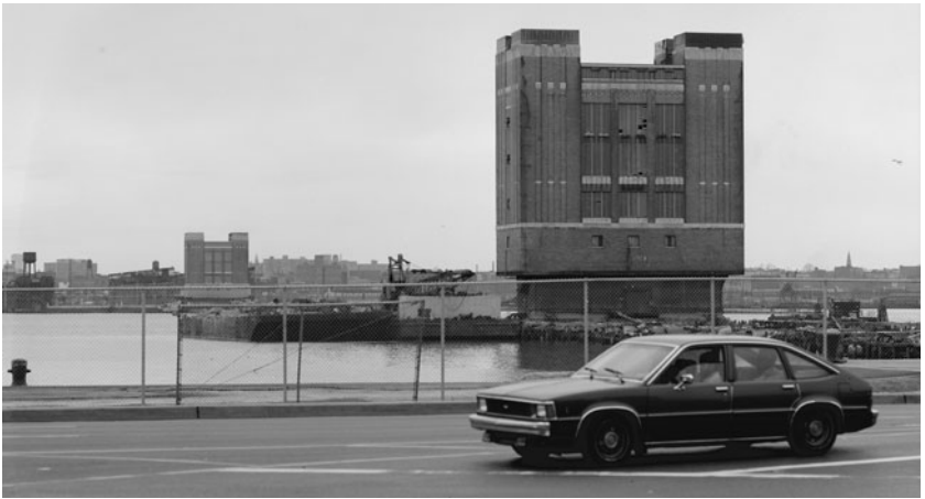
Top: New York river ventilation building, looking east, 1927; bottom: New York river ventilation building, looking west, 1987
