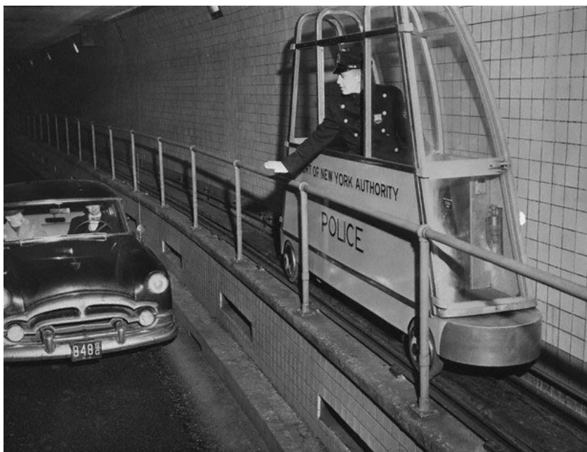
Top: north tunnel, looking east, ceiling removed, 1987; bottom: two-way electric-powered patrol cars tested in 1954
