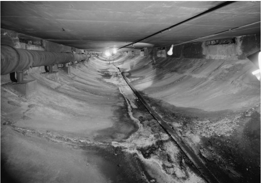
Top: New Jersey river ventilation building, looking west, 1927; bottom: fresh-air duct under roadway, south tunnel, 1987
