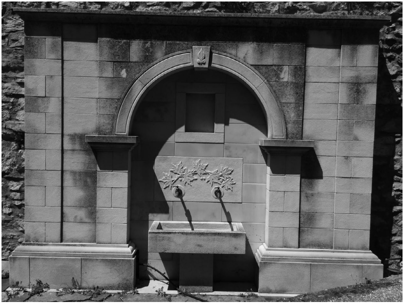
Figure 3.2 A recently restored old fountain in Gonies village
