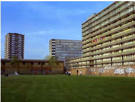
Abb. 22 Mark Lewis, Tenement Yard ( Heygate Estate ), 2002
