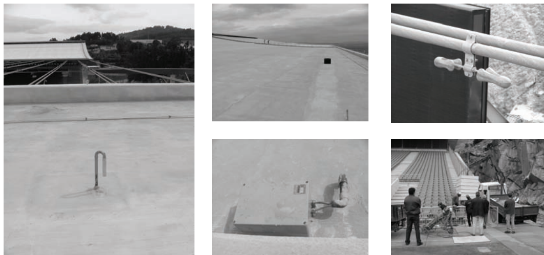
Figure 3.11 Monitoring system on the whole structure
