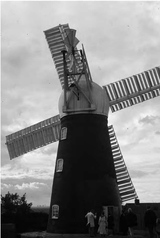
Fig. 11.14. Ellis' Mill, Mill Road. The last of the line of windmills which had stood along the cliff edge since the medieval period. This small tower mill was rebuilt in brick in 1784 and restored by the Lincoln Civic Trust in 1977 (Plate 7.2) (photo and copyright, D Stocker).
