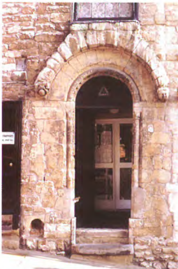
Plate 4.3 Late 12th-century doorway into Nos. 46-7 Steep Hill.
