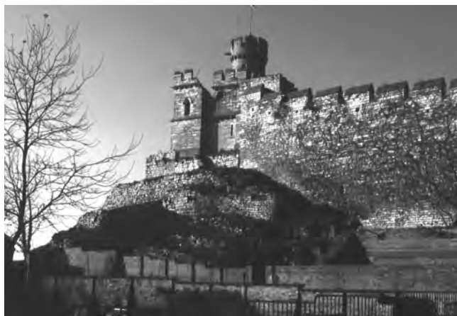
Fig. 9.14. The south-east angle tower of Lincoln Castle (known as the Observatory Tower) from the north-east on its distinctive motte. Both the tower and the wall adjoining it have been greatly restored and little of the original 12th-century fabric is now visible (photo and copyright, D Stocker).
