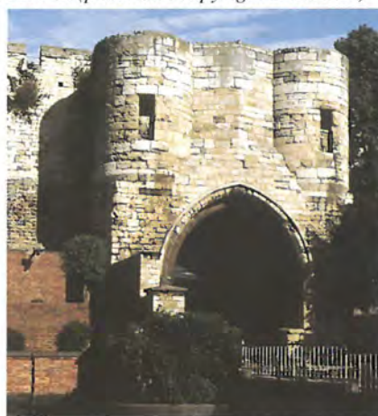
Plate 3.3 East gate of Lincoln Castle. The original 12th-century gate is almost invisible behind the arch and bartizans added, probably, in the 1230s.
