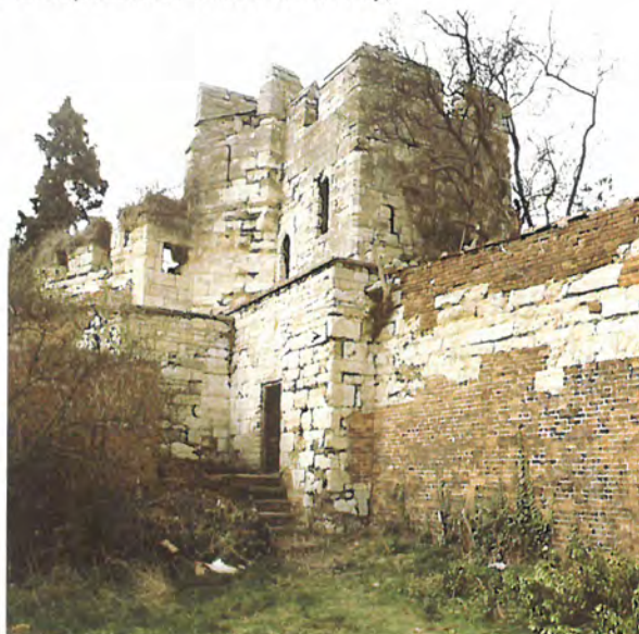
Plate 5.3 Tower on the northern sector of the Close Wall . The tower was the subject of an archaeological recording project and conservation programme in 1992, which demonstrated that it was built in the late 13th century. (photo and copyright City of Lincoln Archaeology Unit)
