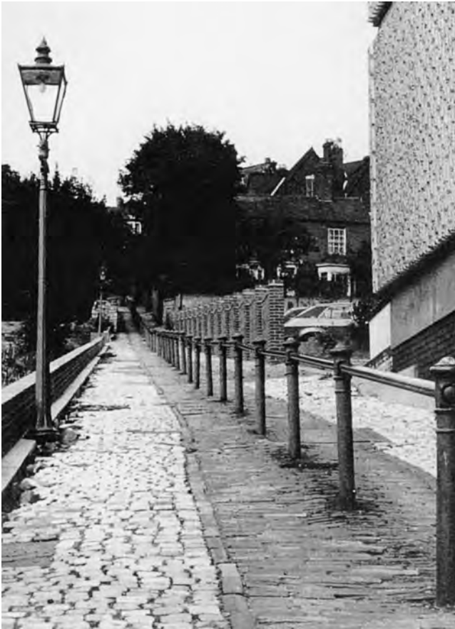
Fig. 11.9. Street furniture looking north along Motherby Hill. These products of the Lincoln foundry industry, still in situ in the 1970s, were the subject of a ground-breaking local recording project by C Wilson (Wilson 1980) (photo and copyright, Catherine Wilson).
