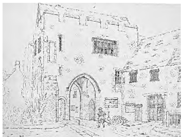
Fig. 9.21. Close gatehouse at north end of Pottergate from the south, a drawing made by Edward Willson made prior to 1815 (London, Society of Antiquaries Ms, 786, portfolio A) (copyright, Society of Antiquaries of London).
