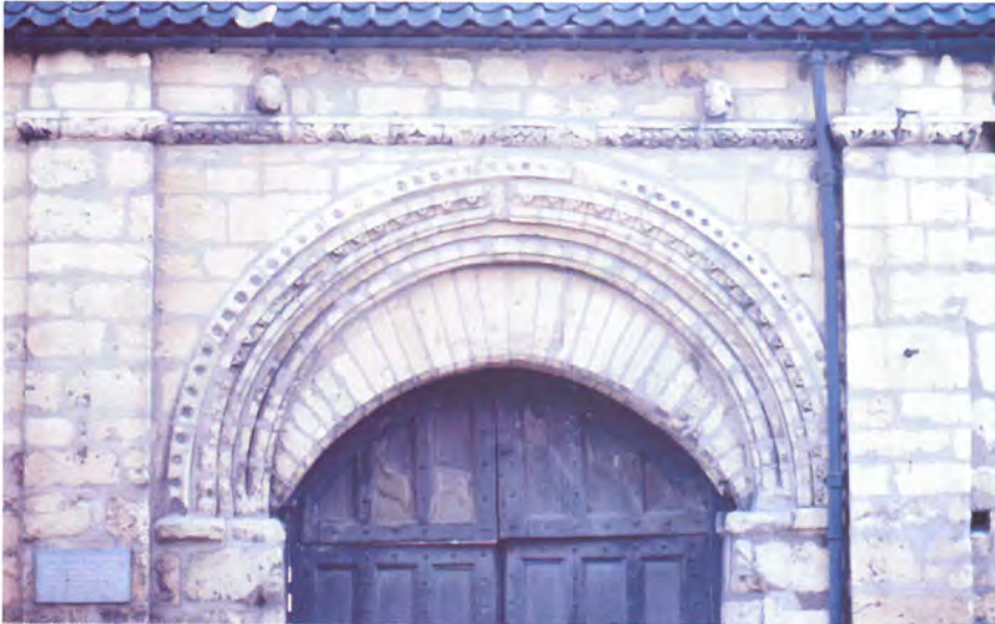
Plate 4.1 West gate-arch of St Mary's Guildhall in Upper Wigford. The arch is the most impressive of the truncated remains of a mid 12th-century town-house of great size and quality, which had connections with the Crown and was the subject of a major archaeological study 1982-6. (photo and copyright D Stocker)
