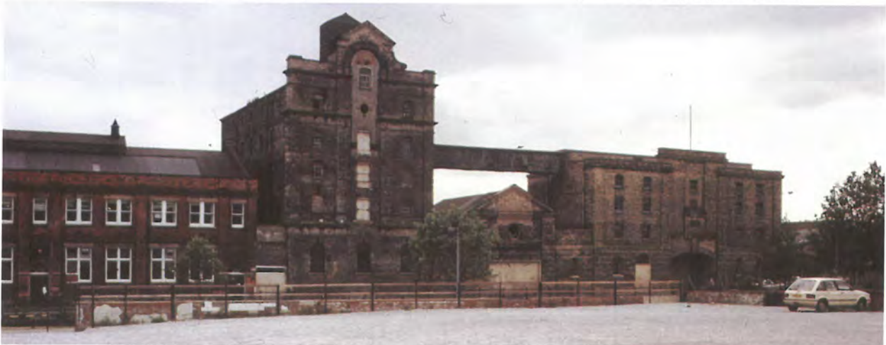
Plate 7.5 Doughty's Mill from the north, across the Witham. The finest of the remaining buildings of Lincoln's once extensive milling industry, the western mill (right) was built in 1863, whilst the eastern 'tower' mill dates from 1891. The building was carefully sited and designed to make maximum use of water transport. (photo and copyright D Stocker)
