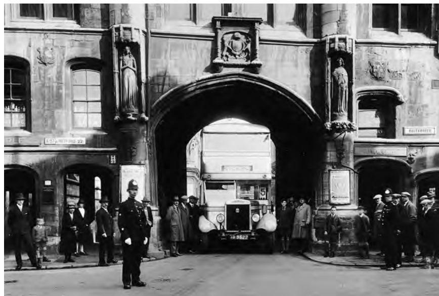
Fig. 10.3. Stonebow from the south – a photograph taken in 1927 to commemorate the first double-decker bus route servicing the new working-class housing estate at St Giles. Co-incidentally it records the condition of the Stonebow's sculpture of c.1520 before heavy restoration (photo and copyright, Lincolnshire County Council, County Library Service, Local History Collection).
