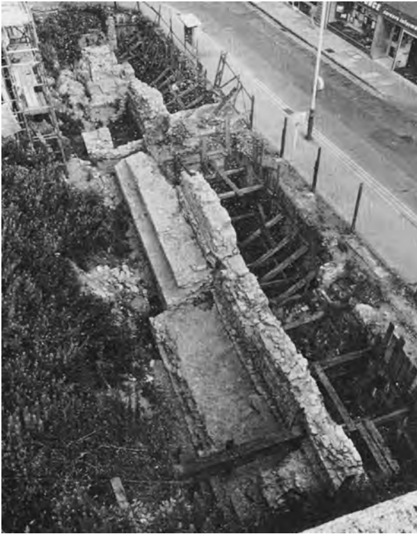
Fig. 10.2. Medieval encroachment over the line of the southern city wall revealed in excavations at Saltergate in 1973 (LIN 73d). The view is taken from the west, looking east along Saltergate. The thick foundation relates to the Roman south wall of the lower city, whilst the narrower walls on top represent medieval domestic buildings facing Saltergate (photo and copyright, English Heritage).
