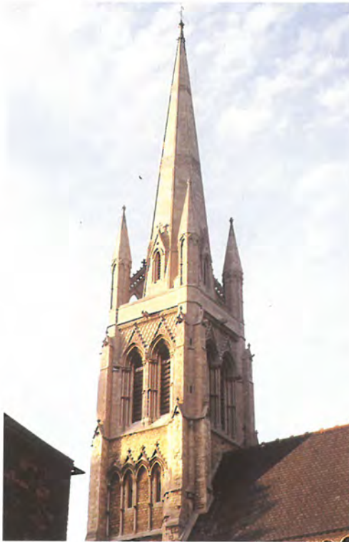
Plate 7.3 The spire of St Swithin's church, the grandest of all the Anglican structures in the city of Victorian date. It was designed by architect James Fowler of Louth and erected in 1884-7 as a memorial to Lincoln ironmaster Joseph Shuttleworth by his son Alfred.
