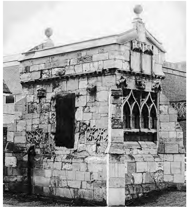
Fig. 10.19. Conduit-head (i.e. the stone container for a water-storage tank) erected in St Mary-le-Wigford churchyard in about 1540, from the north-east. Note the reused architectural fragments, including panels with the Kyme family arms, brought here from the family chapel at the Whitefriars, which was demolished when the friary was dissolved. See also Fig. 9.77 (photo and copyright, D Stocker).
