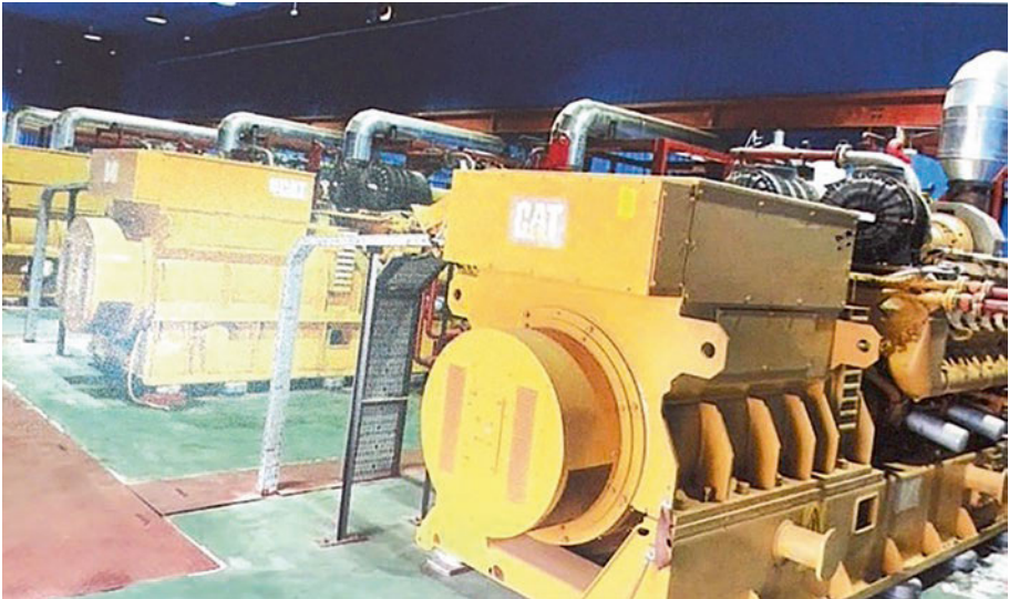
Fig. 10.2 Delta State Oghareki Power Plant Site behind gate
