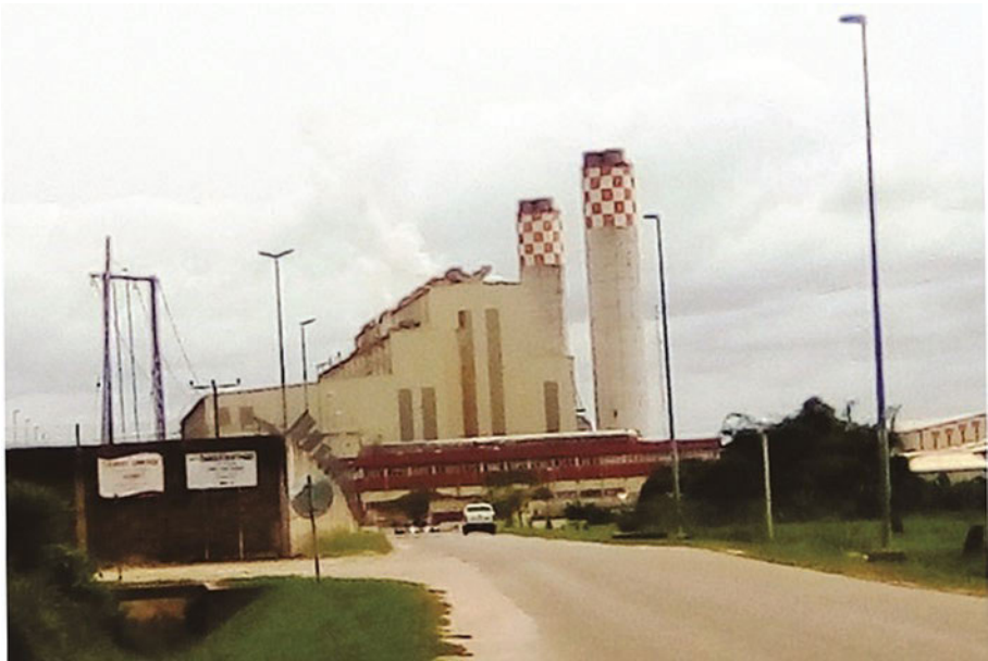
Fig. 4.5 Egbin Power Station
