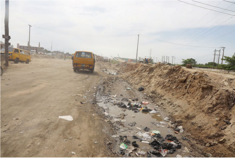
Fig. 9.4 Large portions of the Express Road are still under construction in 2021
