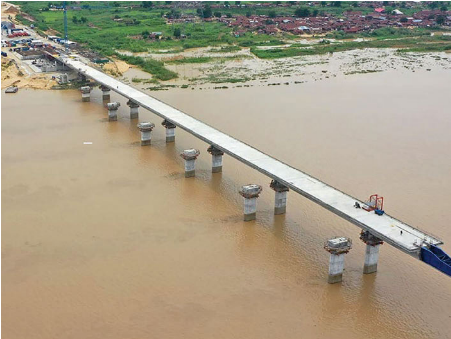
Fig. 4.4 Second Niger Bridge
