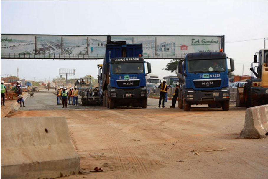
Fig. 9.2 Lagos-Ibadan Express Road during the habilitation contract
