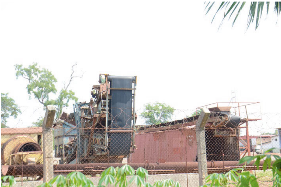
Fig. 4.14 Otukpo Dam Equipment Yard
