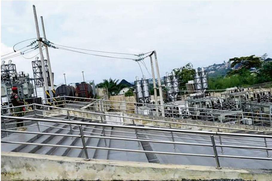
Fig. 4.6 Calabar Power Station
