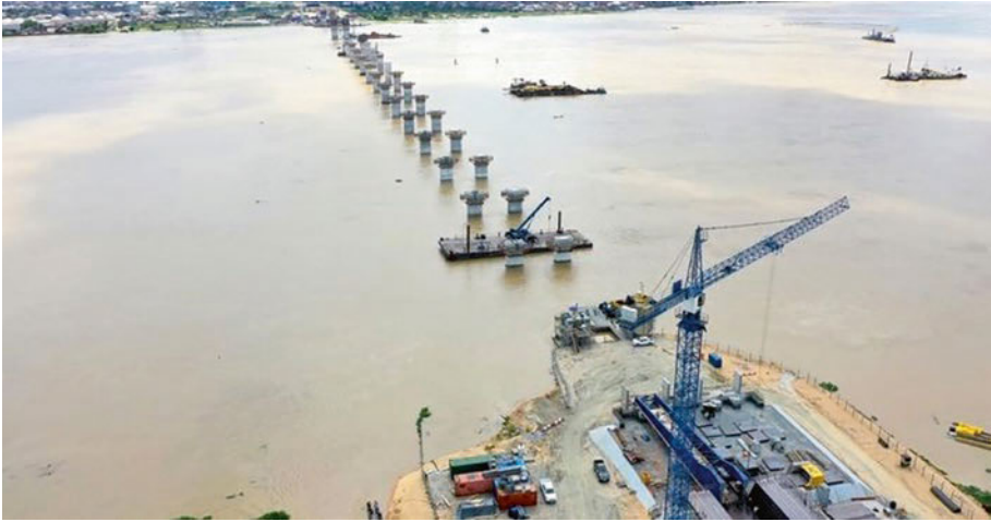
Fig. 7.1 The Second Niger Bridge at 17% completion in 2021
