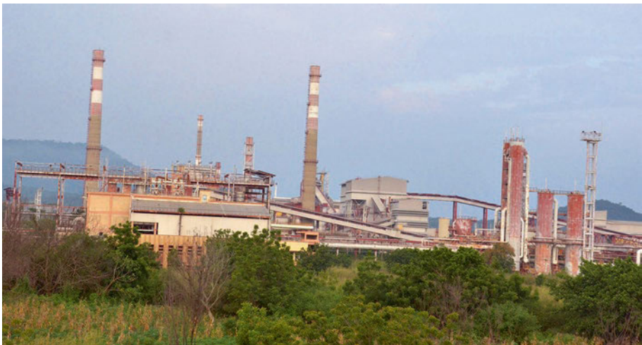
Fig. 4.12 Ajaokuta Steel Plant
