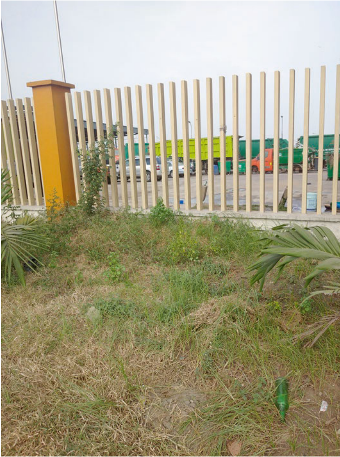
Fig. 4.36 Visionscape Offices after dismantling and being taken over by a company
