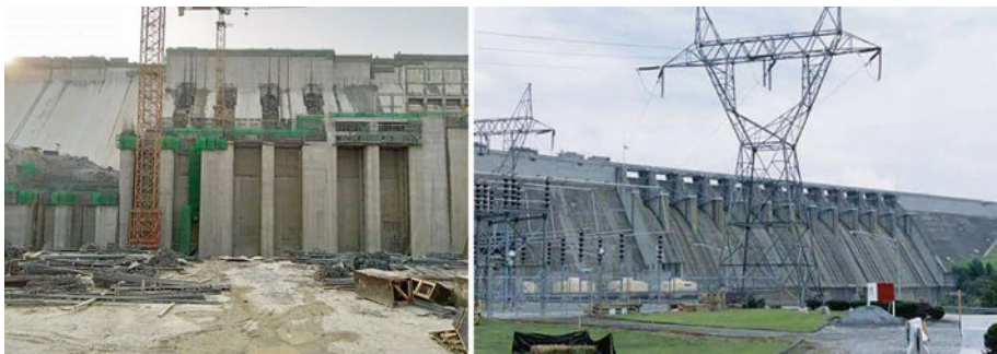
Fig. 10.1 Zungeru construction site in the summer of 2021
