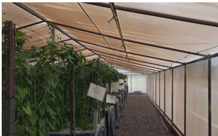
Fig. 14.3 An aeronic screenhouse cooled by showering and misting systems
