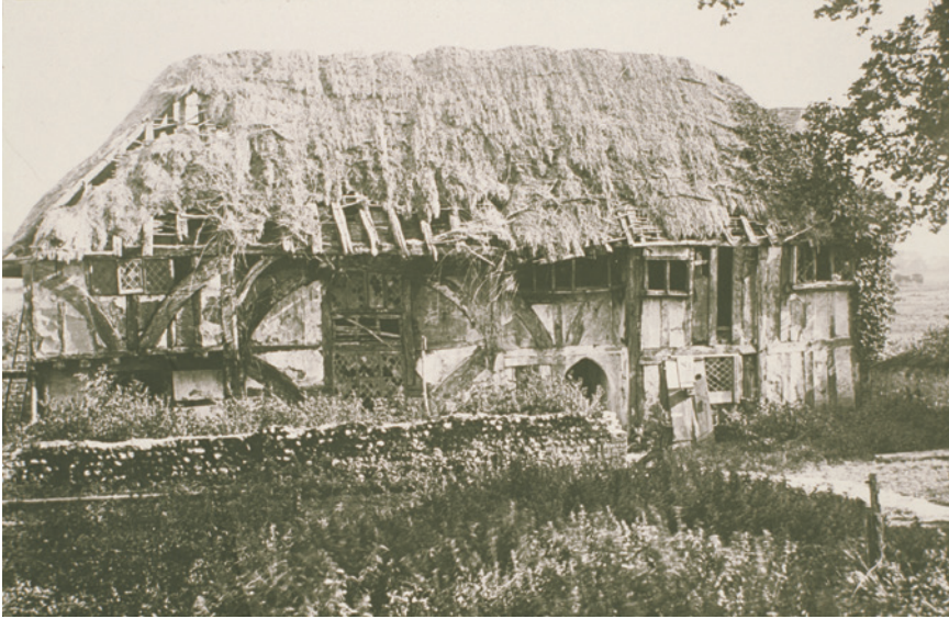
Figure 2.5. Alfriston Clergy House before restoration.
