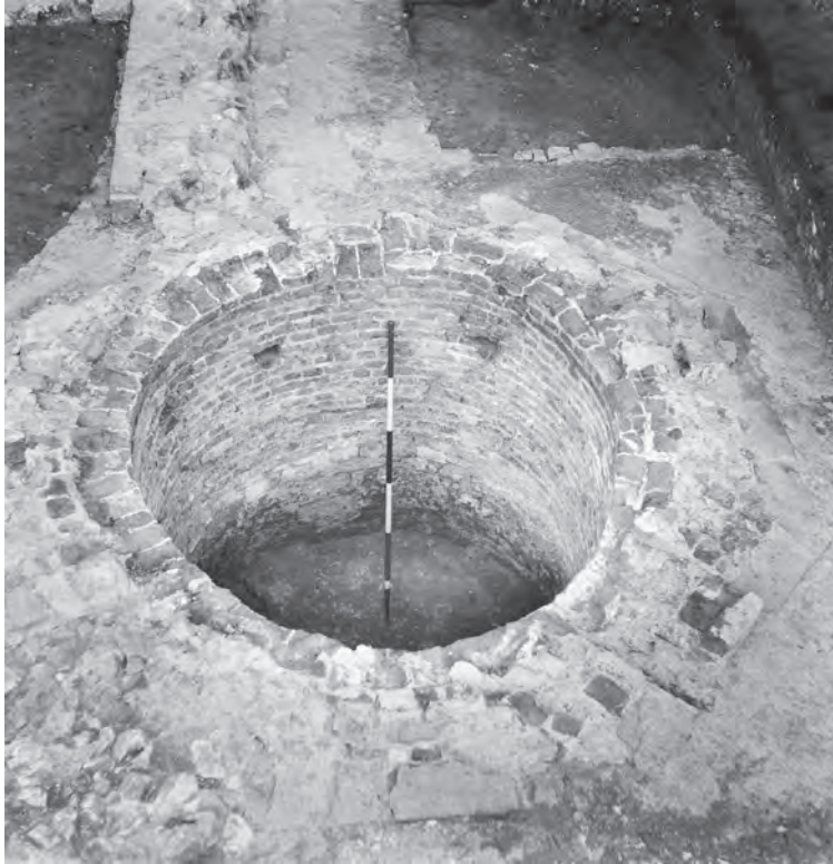
Fig. 16 Nonsuch Palace: Garderobe 1, looking west. Opposed pairs of canted bricks (above and 'below' the ranging rod) indicate the springing of an arch across the garderobe (cf Fig 15).
