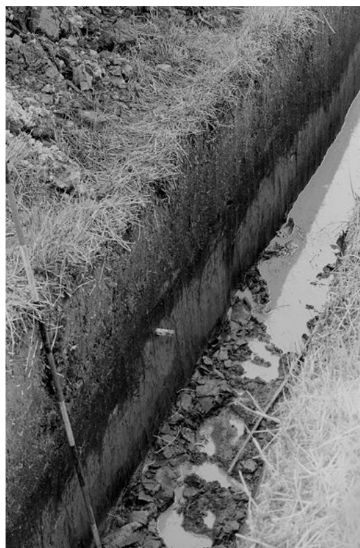
Figure 6.19 East wall of drain A11d/e in the area where grey clay is thickest, view to SSE.
