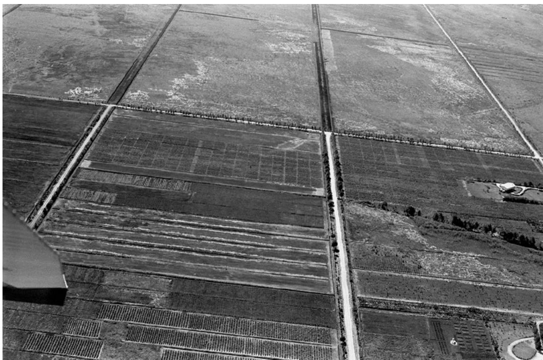
Figure 6.15 Developing the Station drain and road network east of N–S Rd 3, which runs across the middle of the picture.
