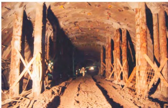
Figure 11. Tree trunks as last resort for shallow NATM tunnel.
