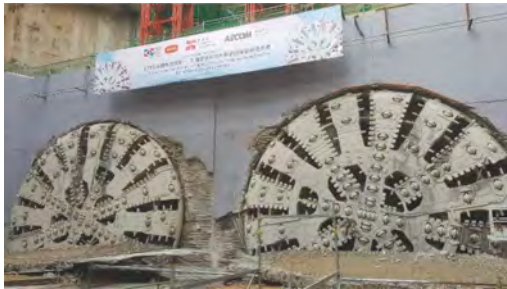
Figure 4. 14m diameter TBMs.
