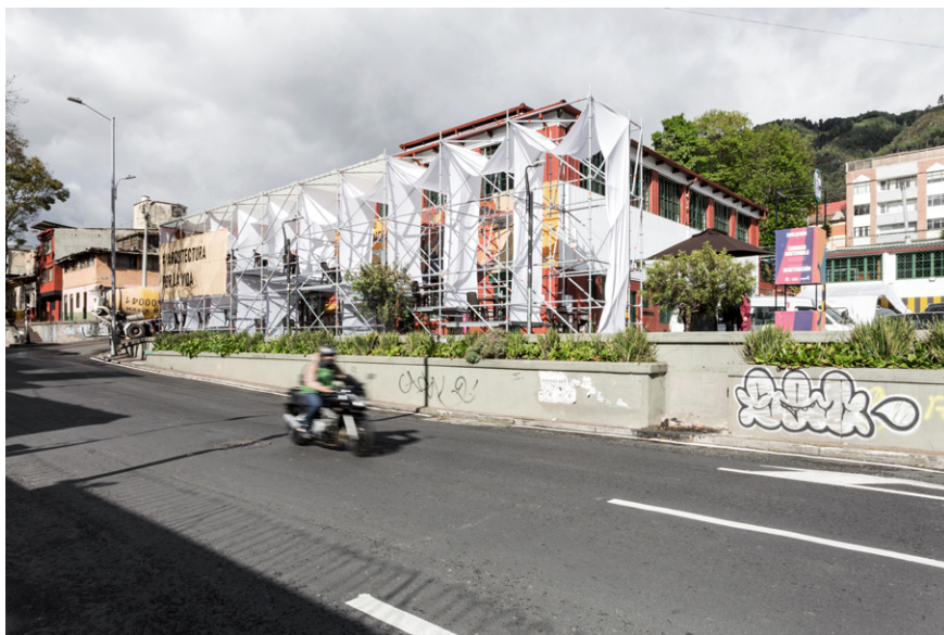
Fig. 5 - Taller Architects, 2020, Vertical Activation, la Perseverancia. Bogotá. Foto: © Pablo Forero.
