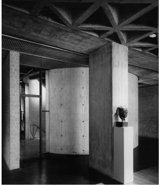
2.27 View of interior looking towards the “silo” drum of the staircase showing the trapezoidal ceiling, Yale University Art Gallery, New Haven, Conn., Louis Kahn (1951–53)
