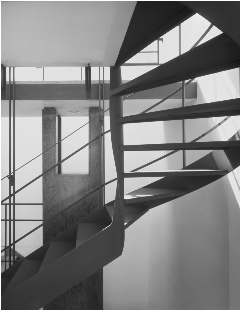
7.11 Artists' Studios for Antony Gormley and Tom Philips, London, 1989, Eric Parry Architects. View of steel spiral staircase to balcony level in Tom Philips' studio
