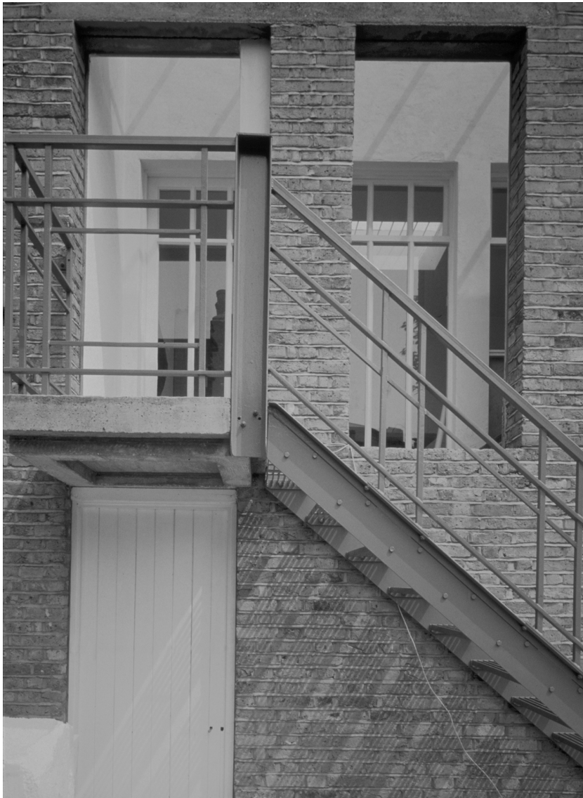
7.13 Artists' Studios for Antony Gormley and Tom Philips, London, 1989, Eric Parry Architects. View of the outside steel and concrete staircase for Antony Gormley's studio
