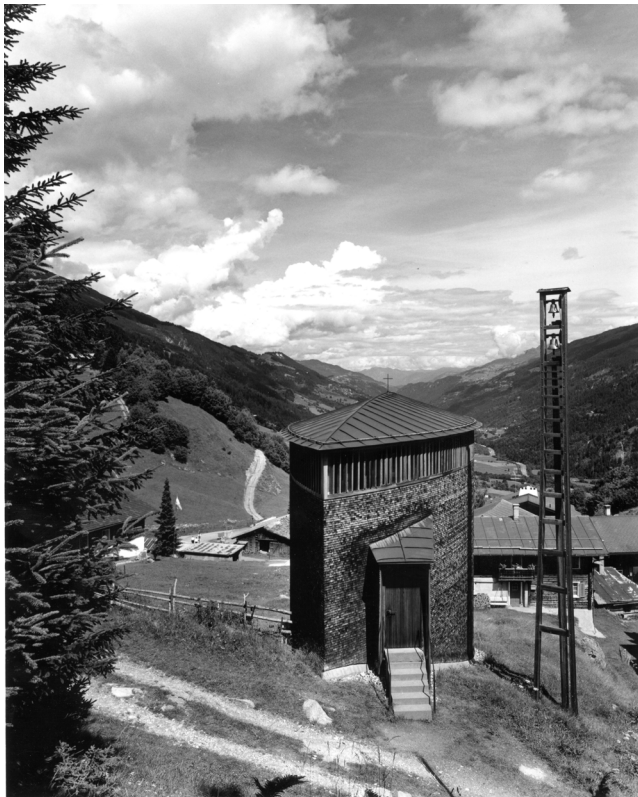
5.16 Caplutta Sogn Benedetg (St Benedict’s Church) 1985–88, Peter Zumthor. View of church from the west showing panoramic views of the valley and mountains beyond
