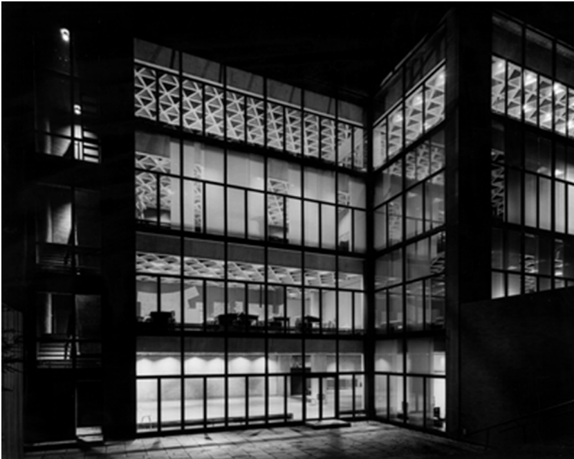
2.31 Exterior view of building during evening with trapezoidal ceilings illuminated, Yale University Art Gallery, New Haven, Conn., Louis Kahn (1951-53)
