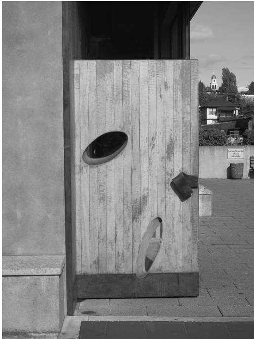
3.13 St Ignatius Chapel, Seattle, 1991–97, Steven Holl Architects. View of the entrance door showing oval shaped glazed openings
