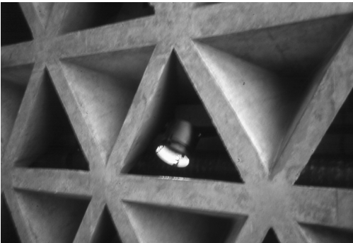
2.28 Detail view of trapezoidal ceiling, Yale University Art Gallery, New Haven, Conn., Louis Kahn (1951–53)
