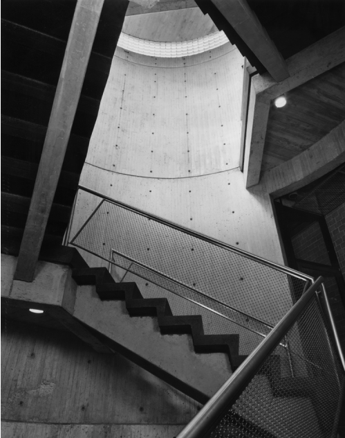
2.30 View of stairwell looking up towards triangular roof-light, Yale University Art Gallery, New Haven, Conn., Louis Kahn (1951-53)
