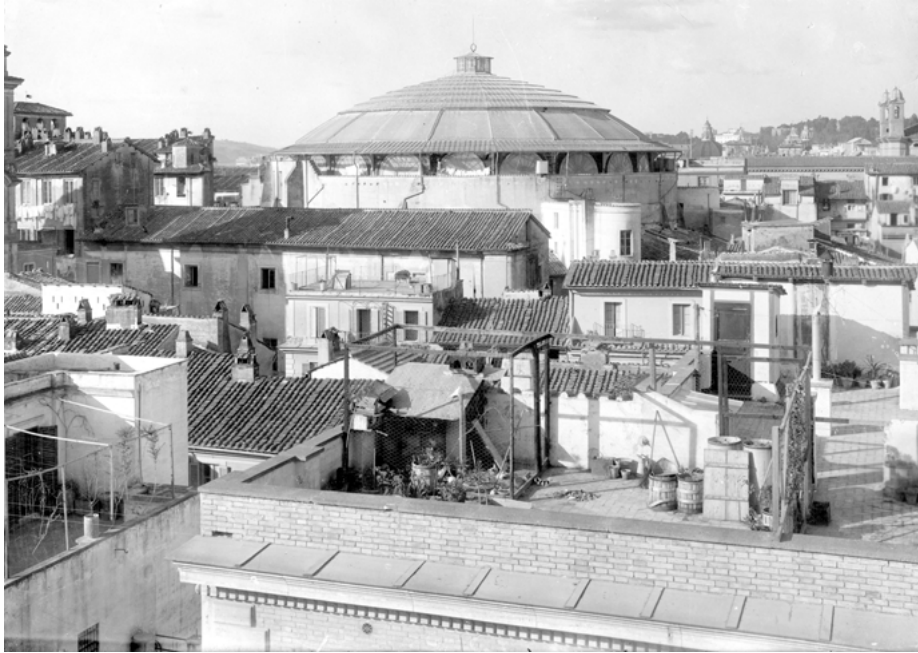
Fig. 7.9: The so-called liberazione of the Augusteo, consisting of the demolition of the later additions. American Academy in Rome, Photographic Archive.
