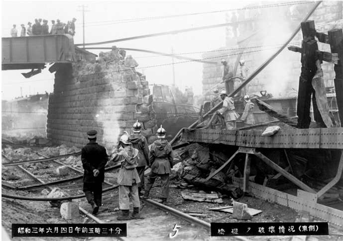
Figure 2.6. The damaged rail bridge after the bombing of Zhang Zuolin’s train just outside Mukden. The caption says in Japanese: “4 June 1928, 5:30 a.m., conditions of destruction of the bridge base (east side).”
