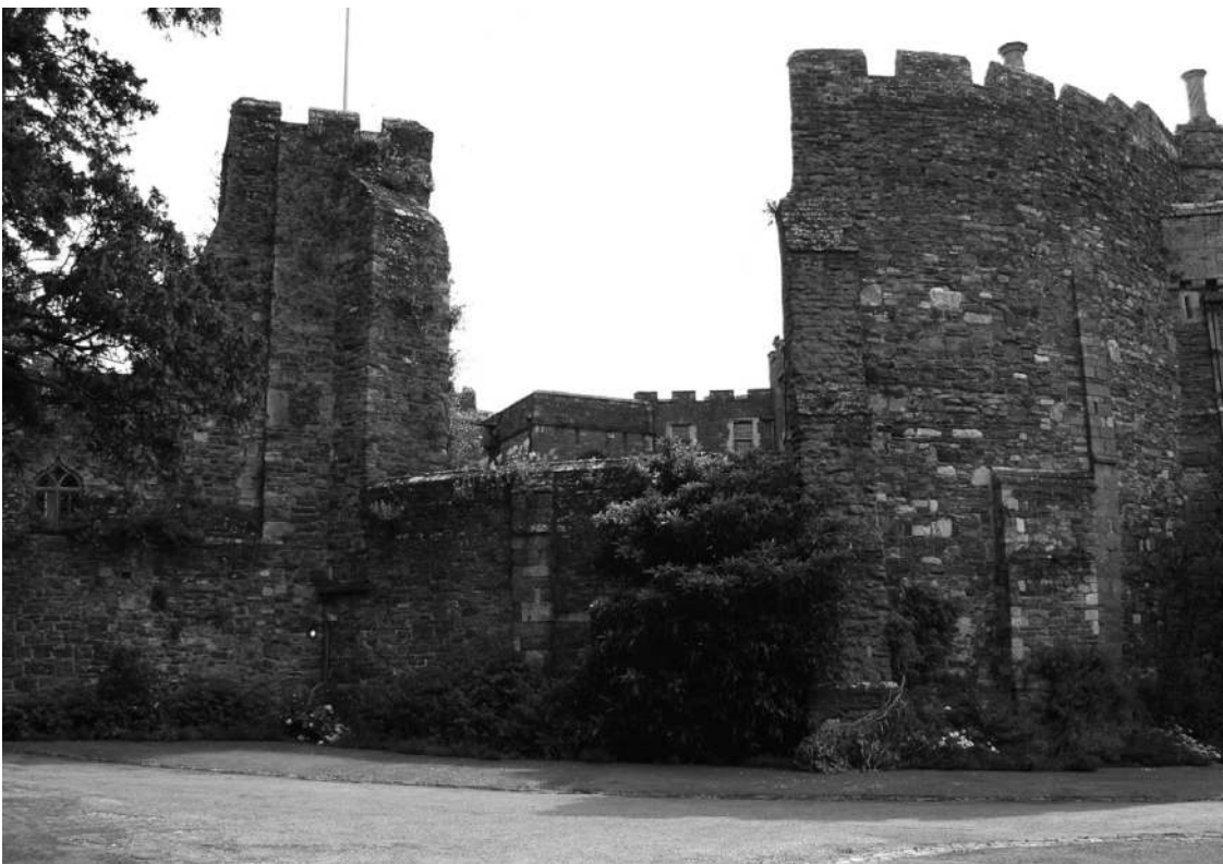
Figure 6. The Civil War damage to the keep
