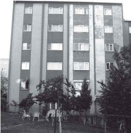
Photo 7 A 5-storey building in Göçmen Konutları ; half repainted, half neglected.
