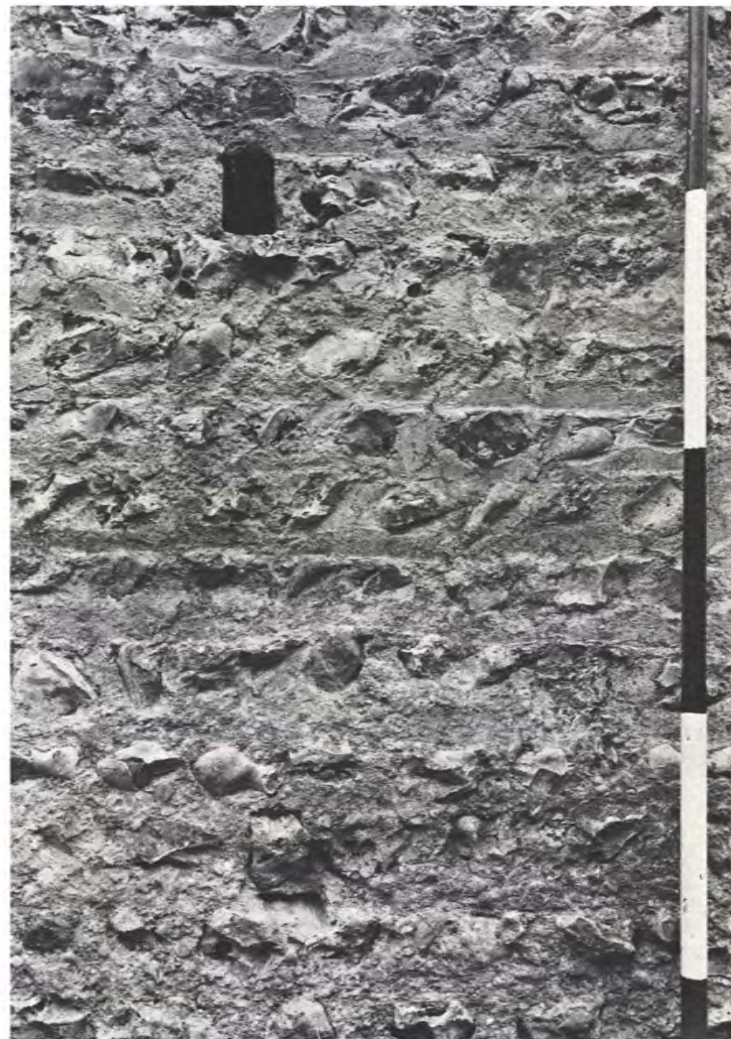
b. The same: detail of pointing of north-west wall and socket (p. 250).
