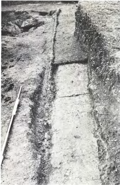
a. Insula XXI, Building 2: Wall 3/4 showing smoothed masonry basis carrying a lath-impression, with clay above: plaster face of Corridor 3 on left (p. 161).
