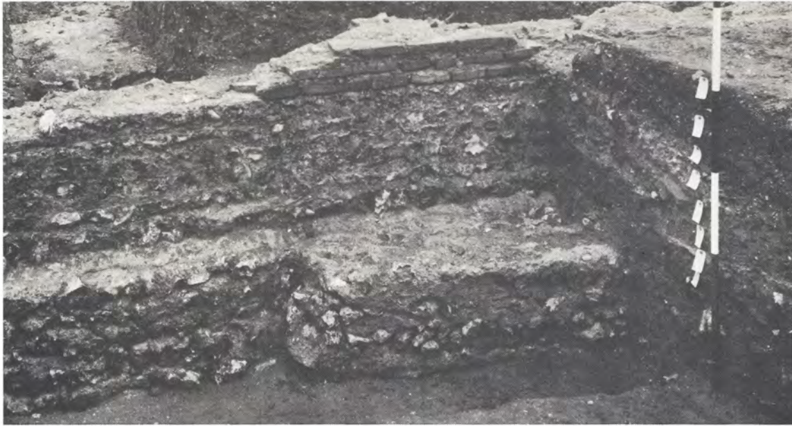
a. Insula XXVIII, Building 1: external face of wall of Room 19, showing triple tile-course and wide foundations (p. 244).
