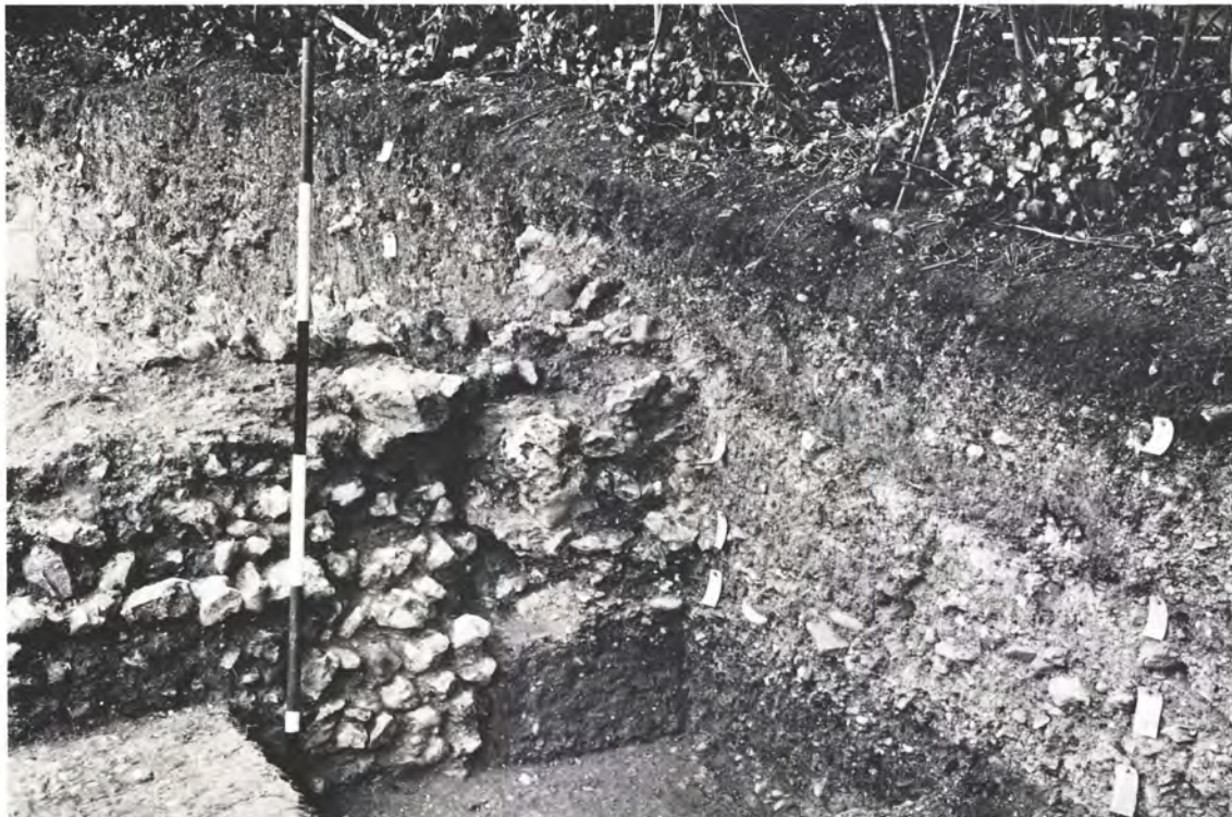
b. Insula XXI, Building I: the blocked door in the north-east wall of Room 3 from north-east (p. 147).
