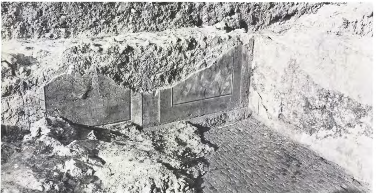
c. Insula XXI, Building 2: painted plaster in situ on south-west wall of Corridor 2 (p. 163).
