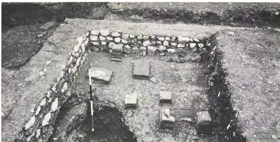
a. Insula XIV, Building 3, Room 1: showing chalk-lined wall and remains of hypocaust (p. 98).
