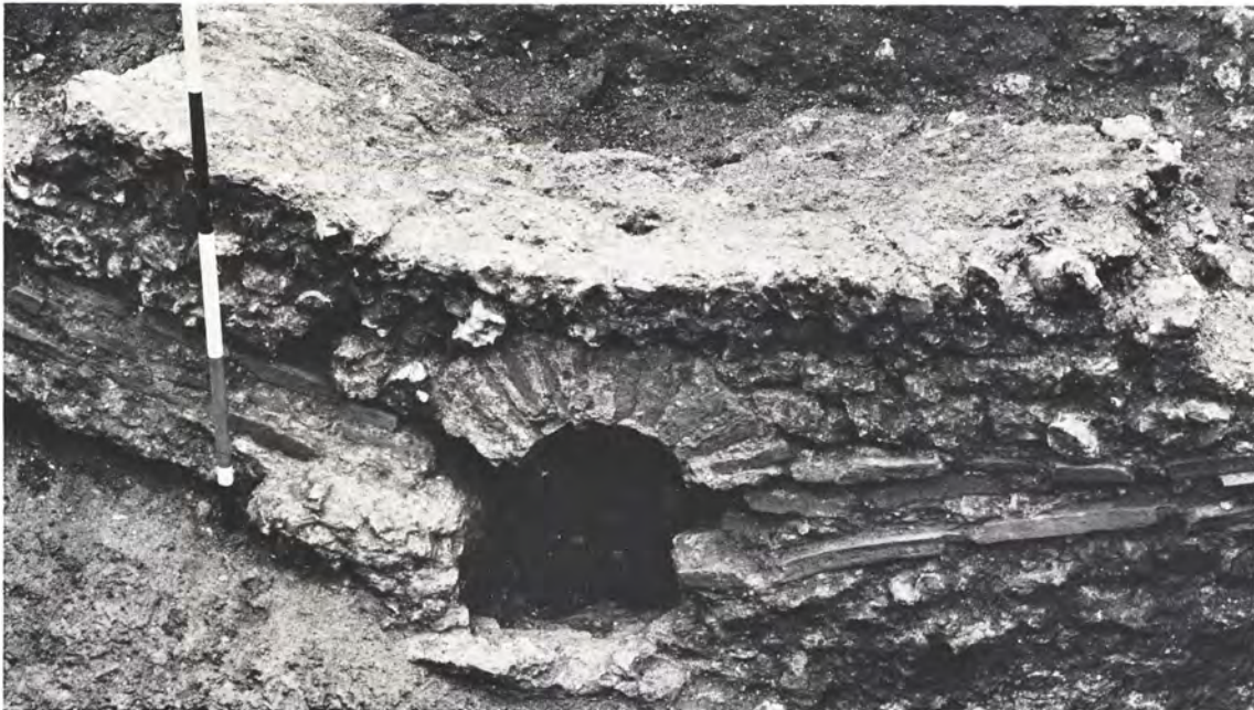
b. Insula XXVIII, Building 1: tile drain-arch through south-east wall of Room 6. The wall has partly collapsed because of tile-robbing along the sewer on its far side (p. 247).
