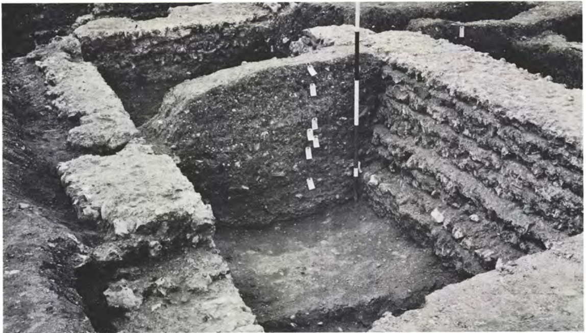
a. Insula XXVIII, Building I, Room 8 showing thick make-up layers above foundations (p. 244) looking south-east. See fig. 107, Section S 1 -T (p. 258).
