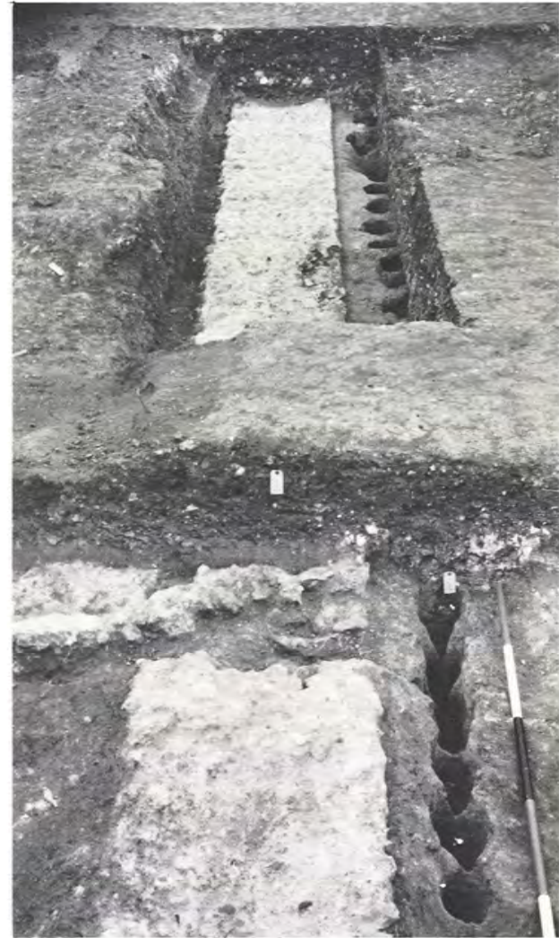
b. Insula XXVII, underpinning of north-east wall of Building 1 running parallel with north-east wall of Building 2, looking north-west (p. 225).
