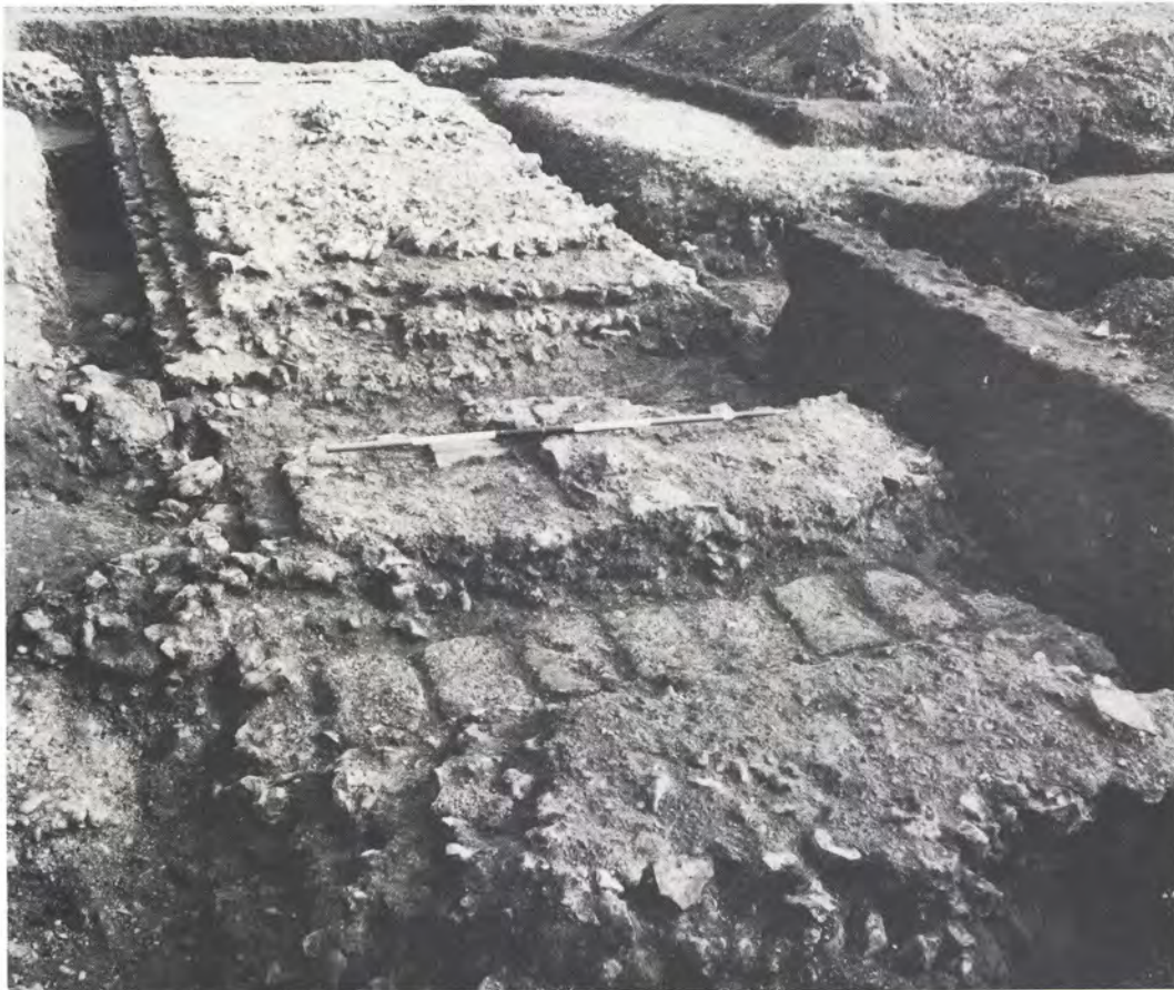
b. The northern Monumental Arch from the south-west showing seating of tile-lined conduit and sewer beyond (p. 75).
