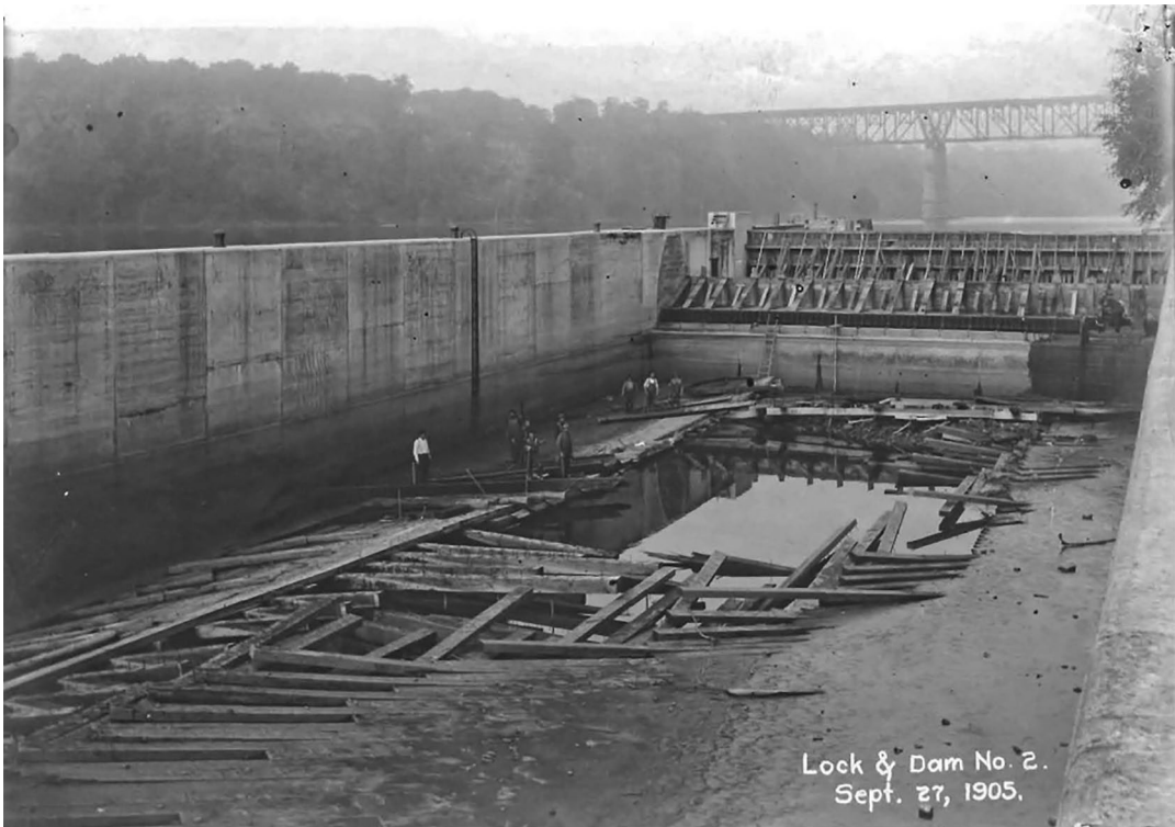
Figure 14.2 Meeker Dam Construction.
