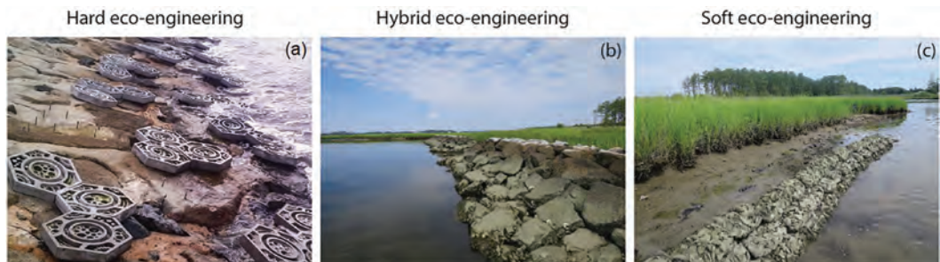
Figure 2 Approaches to ecoengineered shorelines include (a) hard (tile-enhancement units installed along the seawalls at Changi, Singapore), (b) hybrid (rock fillet with saltmarsh in Chesapeake Bay, United States) and (c) soft ecological engineering (bagged oyster shell reef with saltmarsh in Chesapeake Bay).
