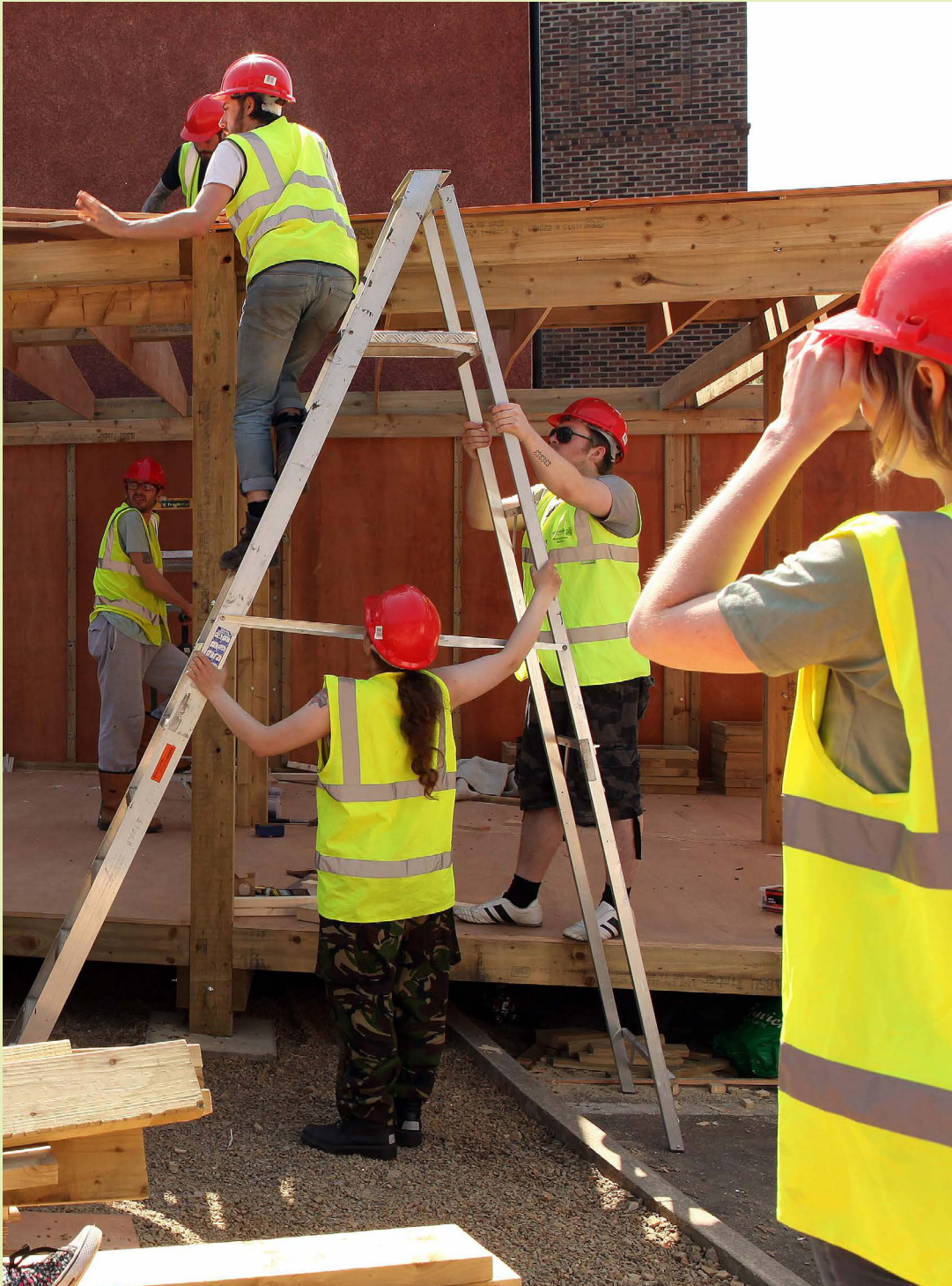
FIGURE III.1.4 Collaboratively lifting the roof panels into place. Photo by John Hipkin.
