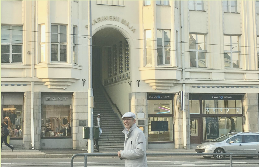
FIGURE III.6.2 Walk through Tallinn. Photo by Prue Chiles.
