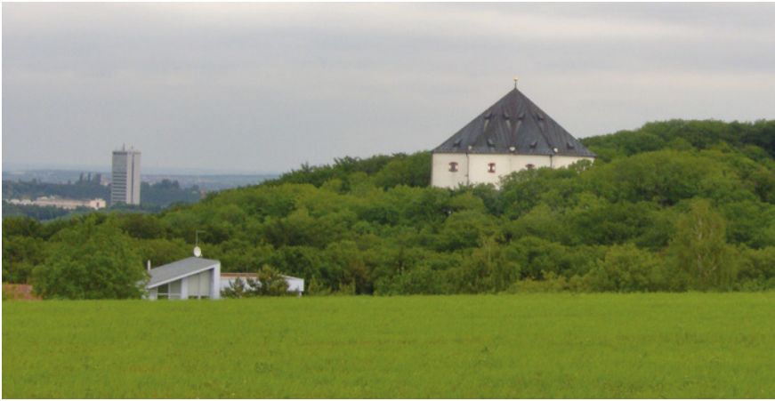
FIGURE 5.61 Prague, hunting-lodge Hvězda (Schloss Stern), built 1555–1560 for Archduke Ferdinand II of Tirol, as seen from the White Mountain.
