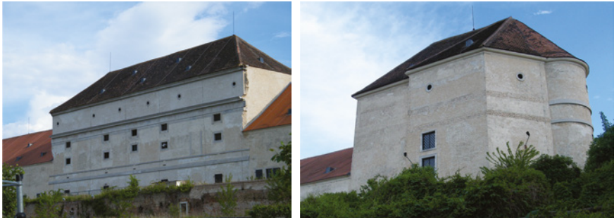
FIGURES 9.105–9.106 North facade and West Pavilion of the Neugebäude, showing remains of the heavy stringcourses originally encircling the whole building.
