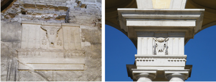
FIGURES 9.32–9.33 The one section of the entablature block which has remained in situ in the Neugebäude, compared to the entablature of the Schönbrunn Gloriette.
