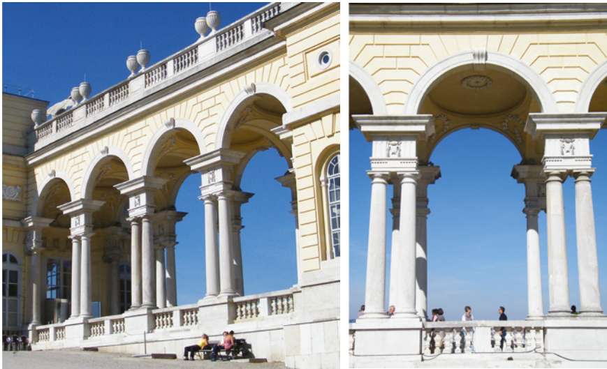
FIGURES 9.34–9.35 The column pairs from the Neugebäude as reused in the Gloriette at Schönbrunn.
