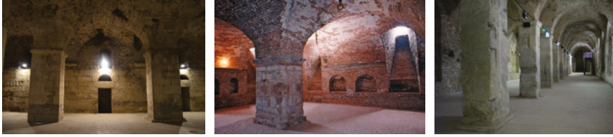
FIGURES 9.57–9.59 The substructures of the Palace at Jülich (9.58) look remarkably similar to those at Split (9.57); but in this case dependence on a more accessible example, such as the third-century cryptoporticus at Reims (9.59) is more probable.
