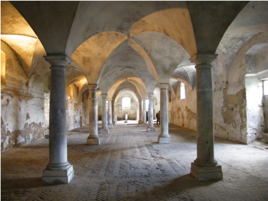
FIGURES 9.24–9.25 The service court of the Neugebäude with the fishponds (on the left); the stable.
