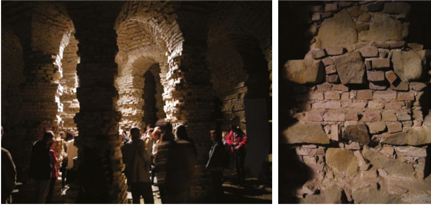
FIGURES 9.78–9.79 A general view of the grotto in the West pavilion of the Neugebäude, and a detail showing its building method and –material.
