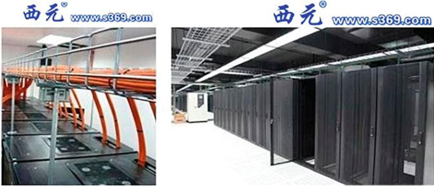
**Fig. 2.67** Ceiling-mounted cabling channels
