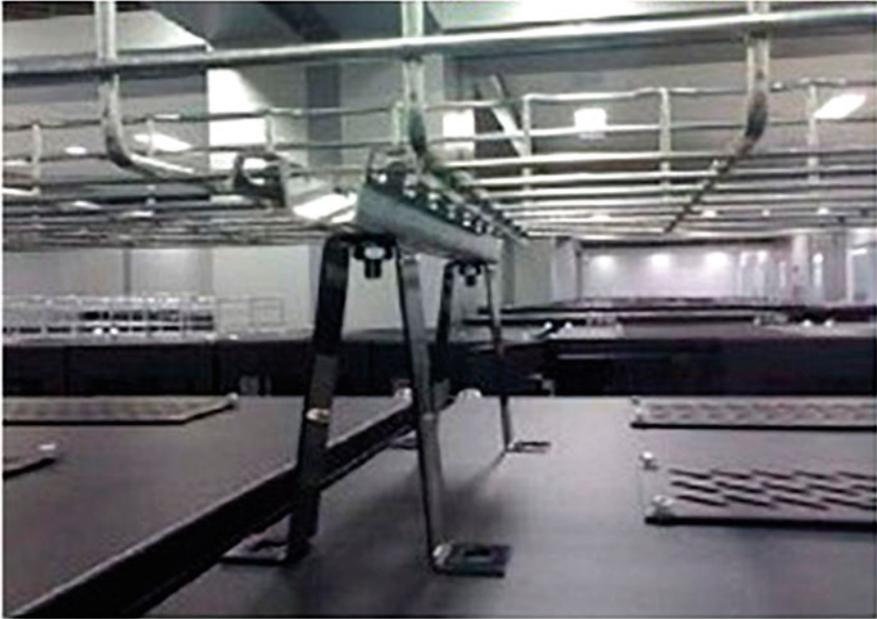
Fig. 2.64 Installation of supporting bridge for rack
