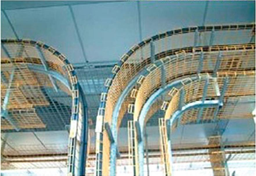
**Fig. 2.63** Layered installation of bridges
