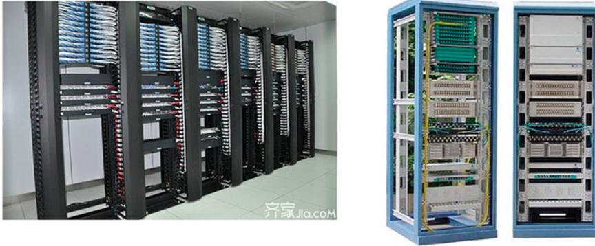
**Fig. 2.8** Cable distribution cabinet in common use
