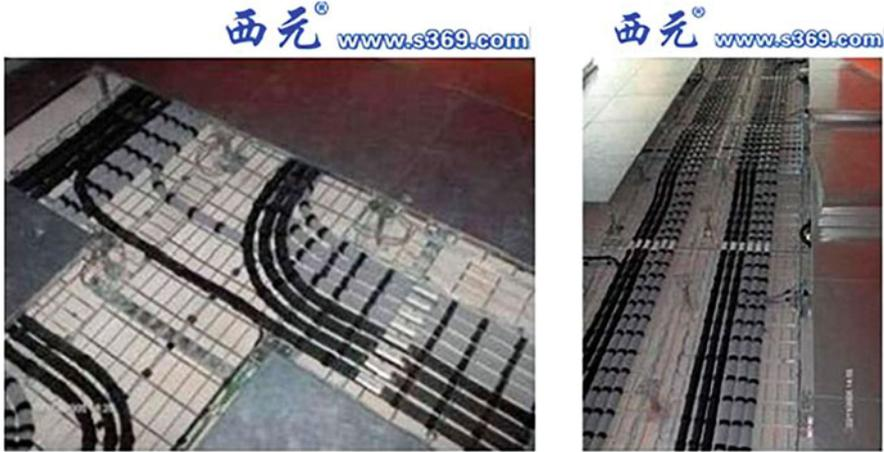
**Fig. 2.66** Cabling channels under the raised floor
