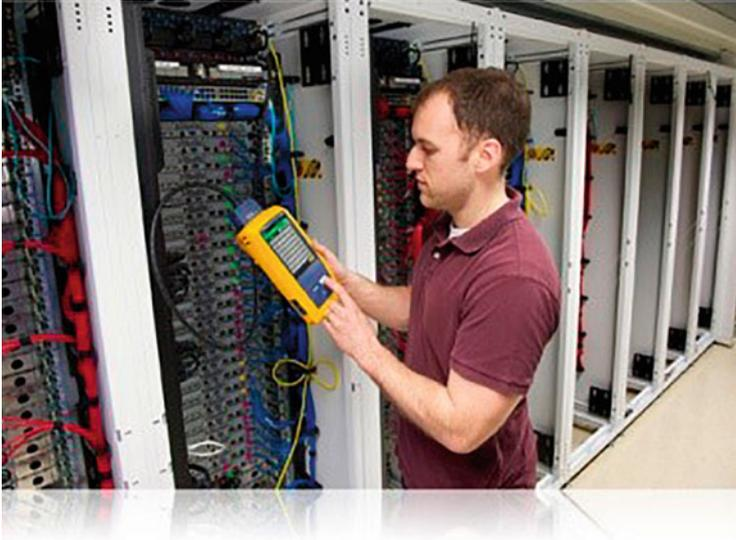
**Fig. 2.51** Troubleshooting using a network tester
