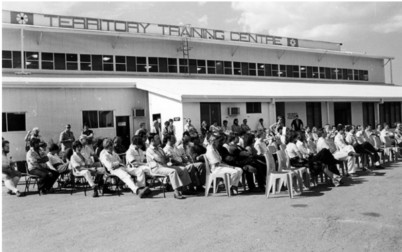
Figure 26. Training Centre, Stuart Park, September 1981.
