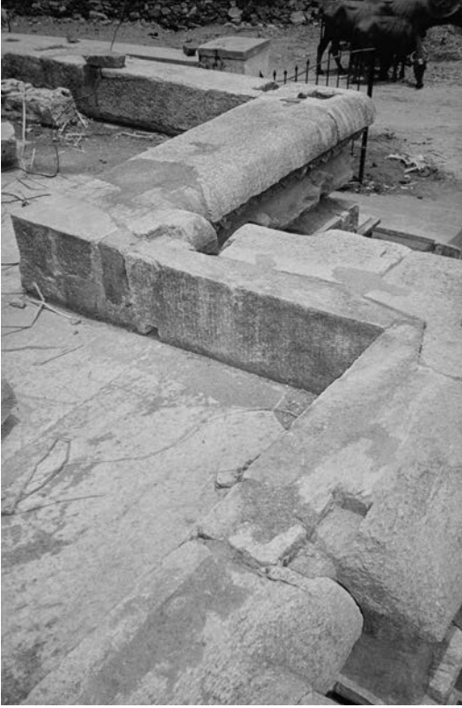
FIGURE 2.6. Subhamaṇḍapa , Jagat. Holes in the masonry suggest the second story may have originally been built of wood. © Deborah Stein.
