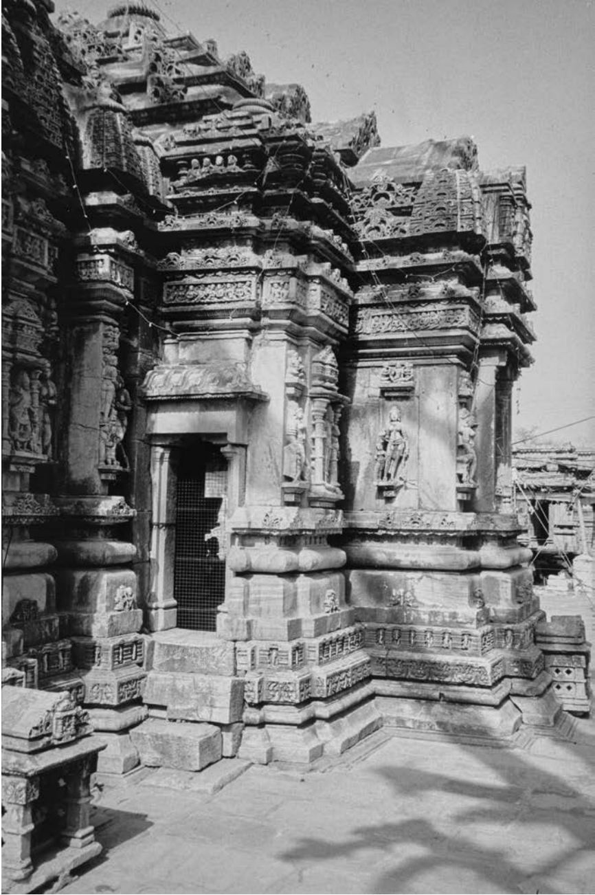
FIGURE 1.6. Door to sanctum on each side allows the bidirectional circumambulation, Ambika temple, c. 960, Jagat. © Deborah Stein.
