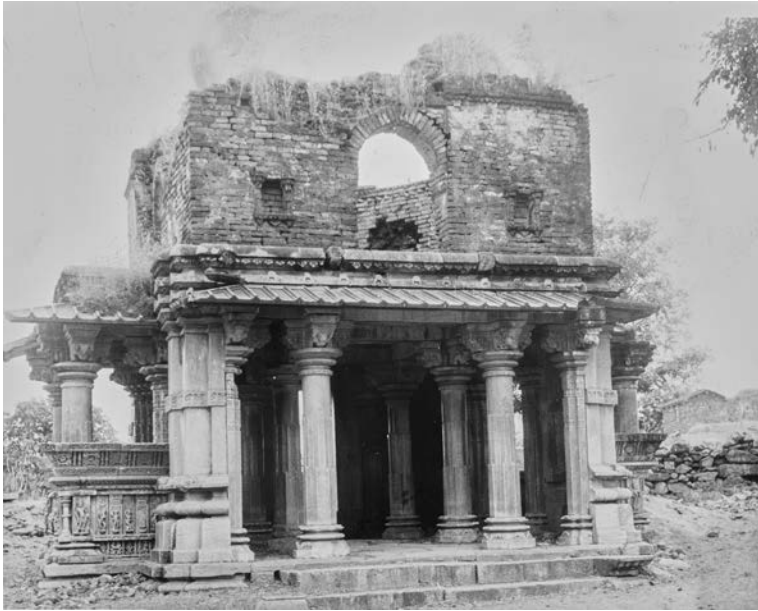
FIGURE 2.5. Śubhamaṇḍapa , archival photo (1950s), building foundation, c. eleventh century; brick layer, c. 1800s–1900s, Jagat. © Archaeological Survey of India (ASI). My sincere thanks to all of the ASI officers who worked together to efficiently provide me with copies of relevant photographs.
