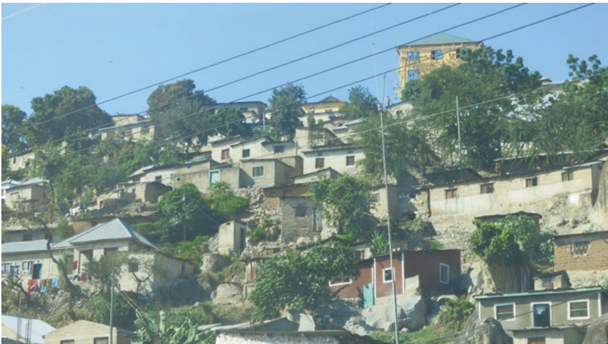
Figure 4. Mwanza City, built on rocks. © Jackline Nyiracyiza Besigye.
