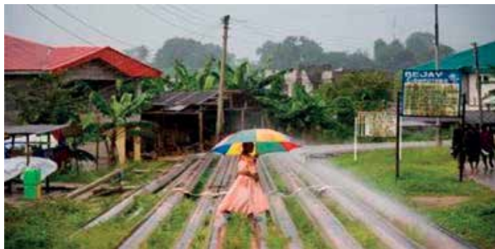
Figure 4. Oil pipelines in Okrika community, Niger Delta [55].
