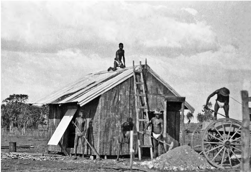
Figure 5.31: Building Aboriginal houses (date unknown).
