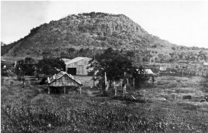
Figure 5.9: View of the early buildings with Arrkuluk Hill in background (date unknown).
