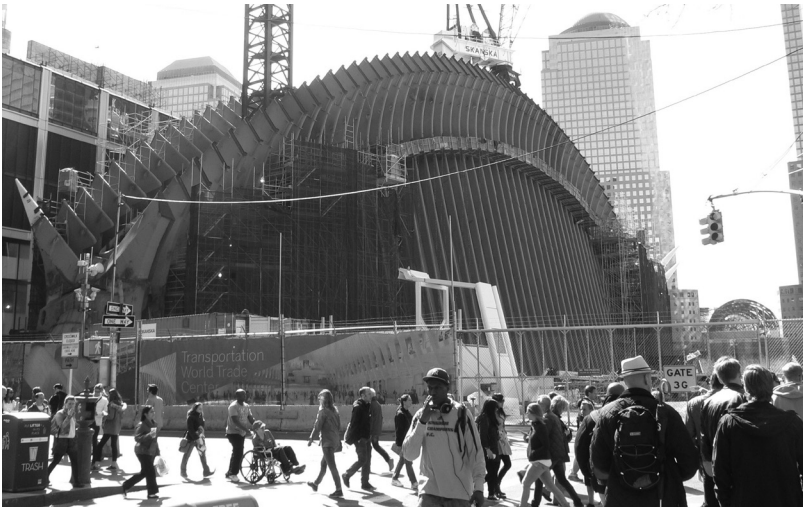
1 Construction site, Ground Zero, May 2014
