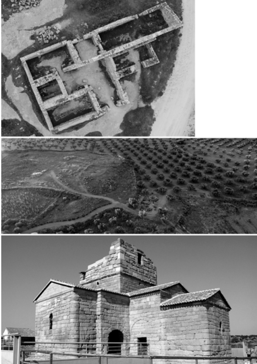
Fig. 16.5 Sacred architecture in the territory of Toledo: a) St. Pedro de la Mata church; b) Guarrazar; c) St. Maria de Melque church. © Isabel Sánchez Ramos and Jorge Morín de Pablos.
