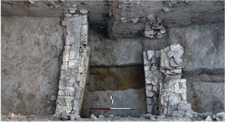
Figure 8.4 The Islamic-period Madjān Canal from above, showing the well-constructed retaining walls. Source: author
