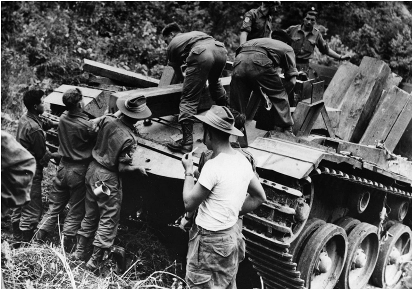
Defence in depth was vital in case of a Chinese breakthrough. Here men from 2RAR unload timber baulks to construct bunkers, most likely on the Hook.
