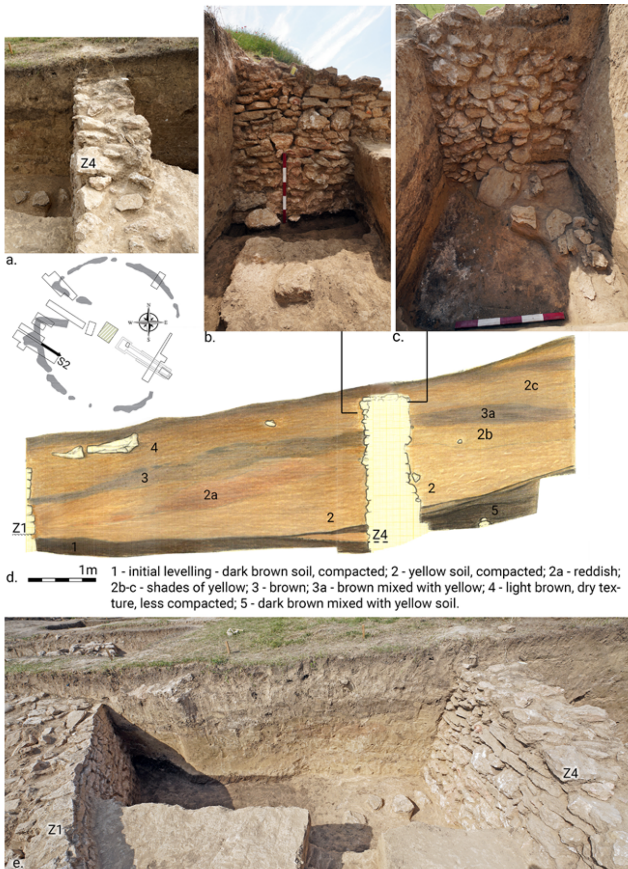
Figure 66. Retaining wall Z4 in S2, behind the krepis , in the western sector.
