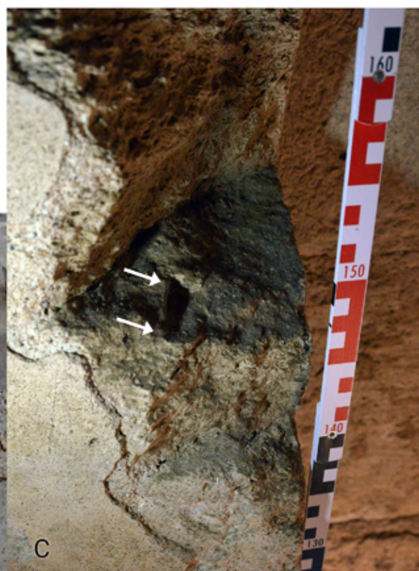
Figure 124. Entrance in the funerary chamber seen from dromos I . Cracks and splits in the lintel area due to weight discharge.
