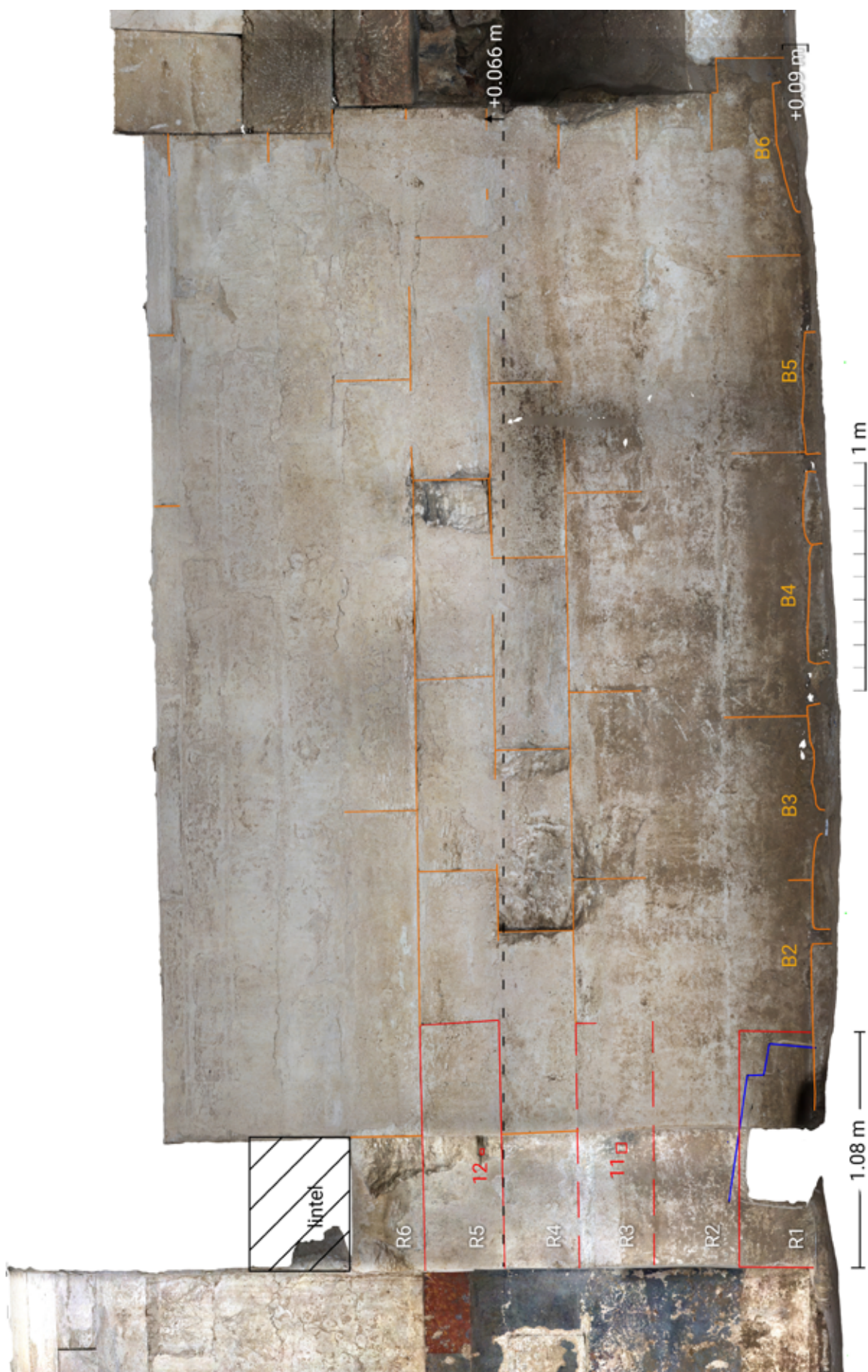
Figure 126. Dromos I , orthophoto of northern wall; orange lines – plinths and ashlars' joints visible in the areas where the plaster fell; red – T-shaped blocks common with the funerary chamber; 11, 12 show the orifices in the entrance; with blue – threshold block; dashed line – an ideal horizontal line.
