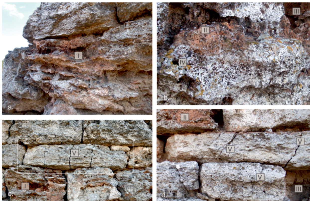
Figure 88. Socle, the northern face: a) example of alveolisation on AB corner dimensioned stone block row 8; b) biochemical weathering; c, d) degradation and alteration of stone: I – alveolisation, II – limonite deposition, III – loss of material; IV – biological crust; V – cracks (photos V. Cetean, Al. Teodor).
