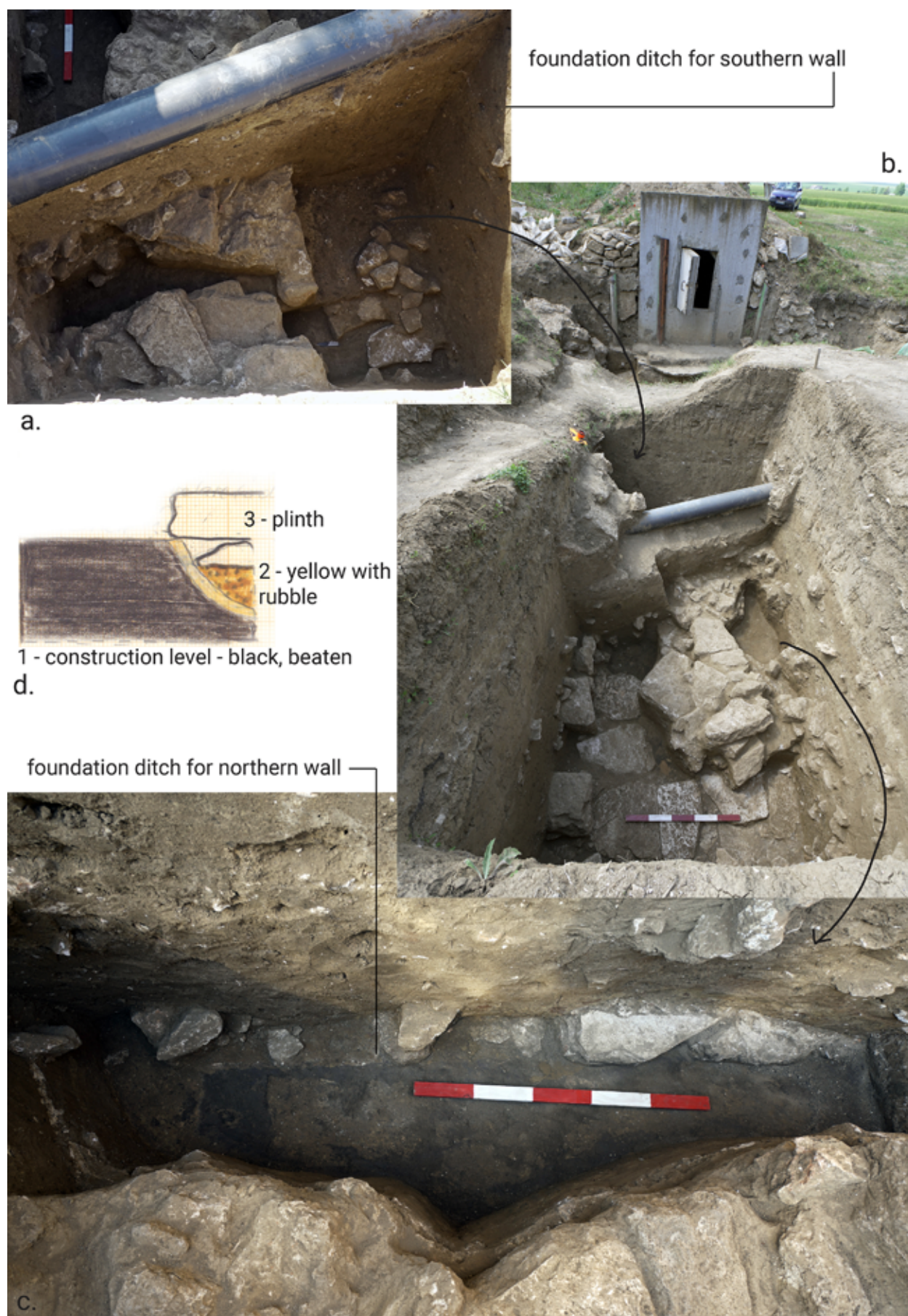
Figure 147. Trench S8, foundation ditches for dromos II walls, slightly deepened in the construction level.
