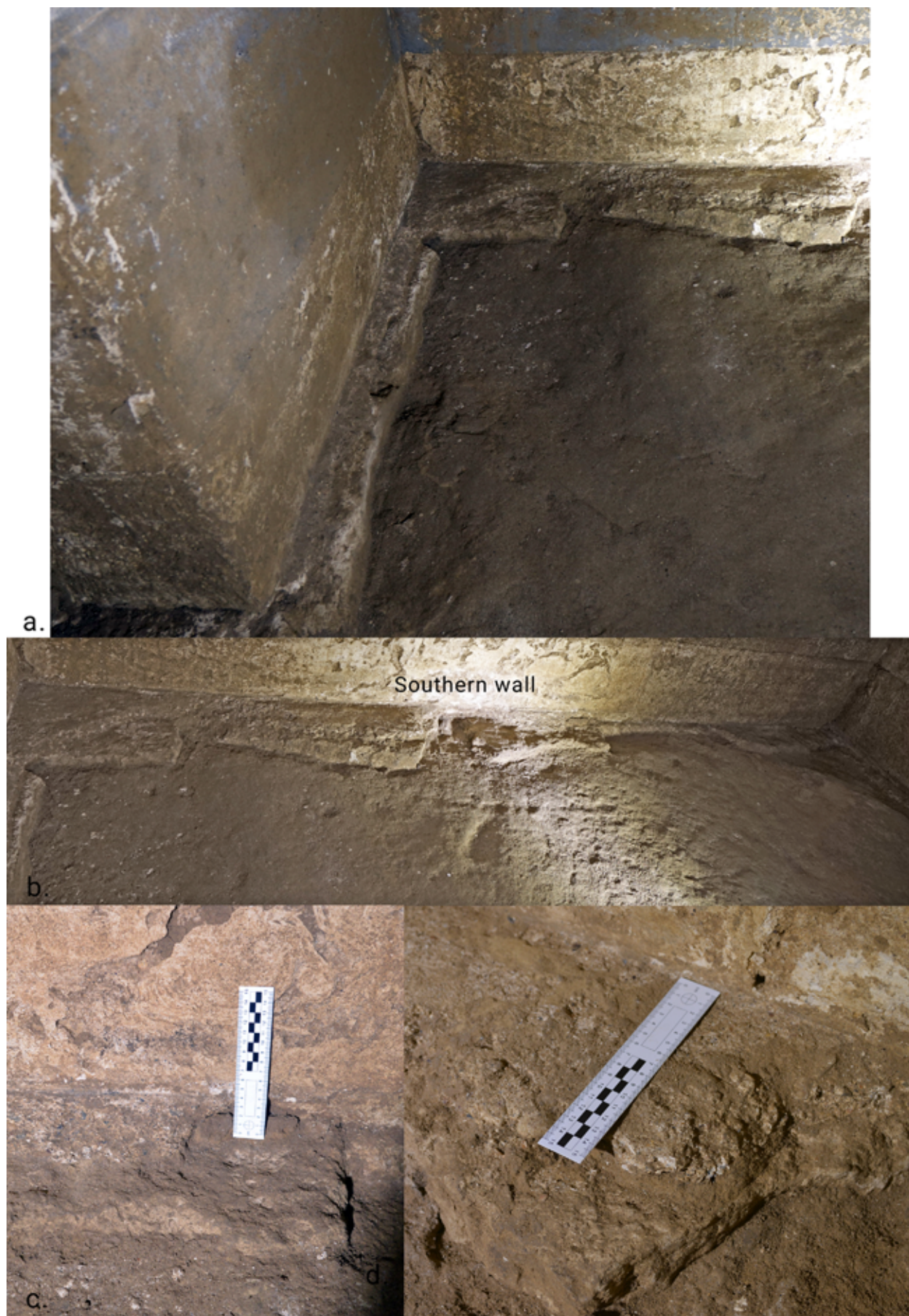
Figure 106. Wall plinths covered with plastered: a) south-eastern corner; b-d) southern wall.
