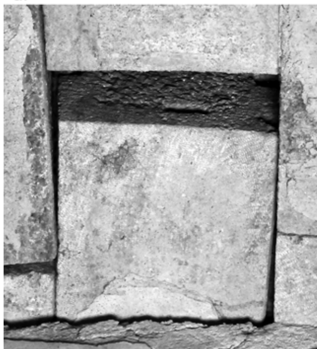
Figure 103. Funerary chamber vault intrados : a) moved voussoirs above the entrance; b) detail with the orifice of a clamp and anathyrosis ; c) fine carving of the intrados blocks.
