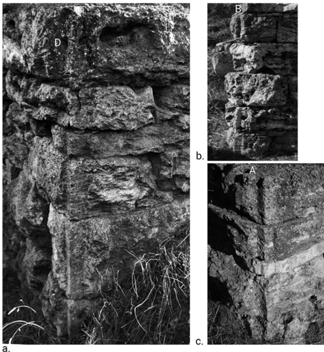
Figure 77. Socle, corners with drafted margins.
