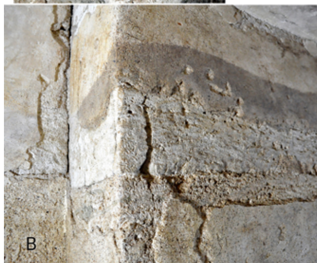
Figure 124. Entrance in the funerary chamber seen from dromos I . Cracks and splits in the lintel area due to weight discharge.
