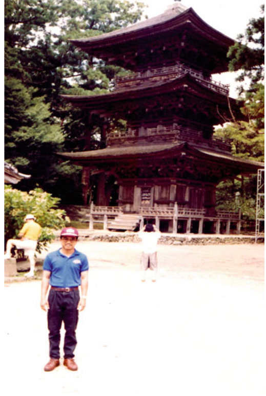
Fig. 8.43 Nakajo Temple, Niigata, Japan. Photo by Arba'at Hassan
