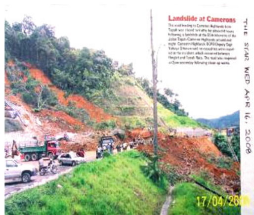
Fig. 8.54 Landslide along highway, Malaysia. Photo by Arba'at Hassan
