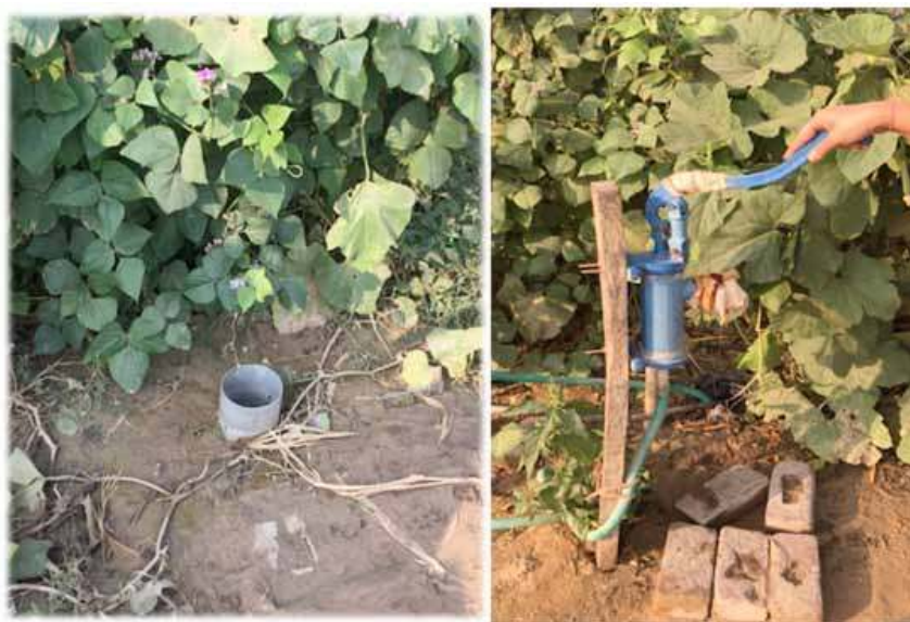
Fig. 24. Photos of Bhungroo Water Storage Opening (Left) and Water Pump (Right). Copyright © 2019 Courtesy of Peggy Ann Spitzer.
