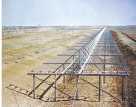
(a) Part of the master transmitter antenna at Lake Kickapoo, Texas, contributing to the AFSSS until 2013. (Public domain image, https://commons.wikimedia.org )
