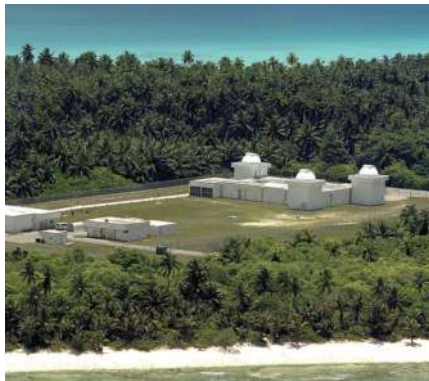
(a) The Diego Garcia site, as one of three GEODSS sites, consists of three Cassegrain telescopes and is located in the Indian ocean. (Public domain image, https://commons.wikimedia.org )
