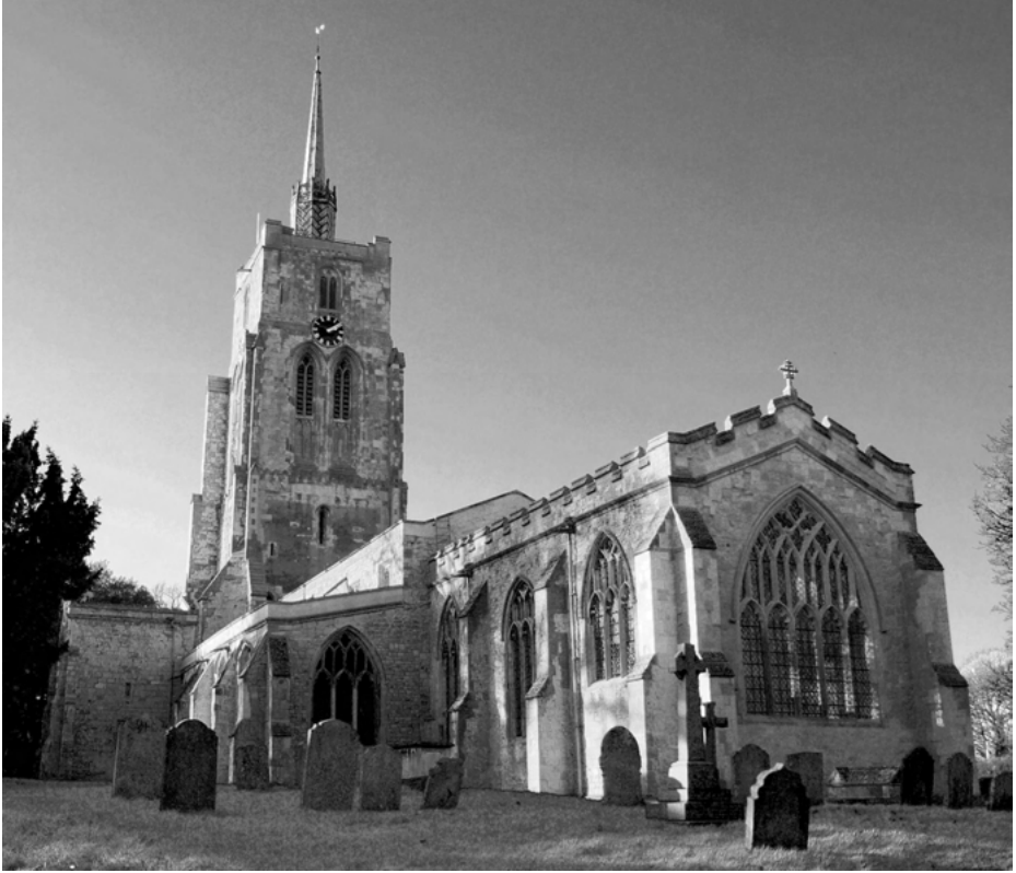
Fig. 3.14: Exterior view of Ashwell St Mary, Ashwell, Hertfordshire. The evidence suggests that masons were working on the building when the storm occurred or shortly after. One possibility, therefore, is that the unfinished building was damaged by the storm. Photograph by the author.
