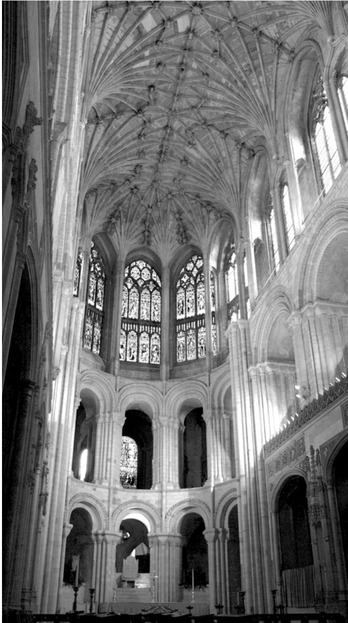
Fig. 3.13: View of Norwich Cathedral's clerestory showing the stylistic disjuncture between the lower Romanesque arches supplanted by later Gothic arches above – a tangible result of the storm of 1362 and the repairs required in its aftermath. Photograph by the author.
