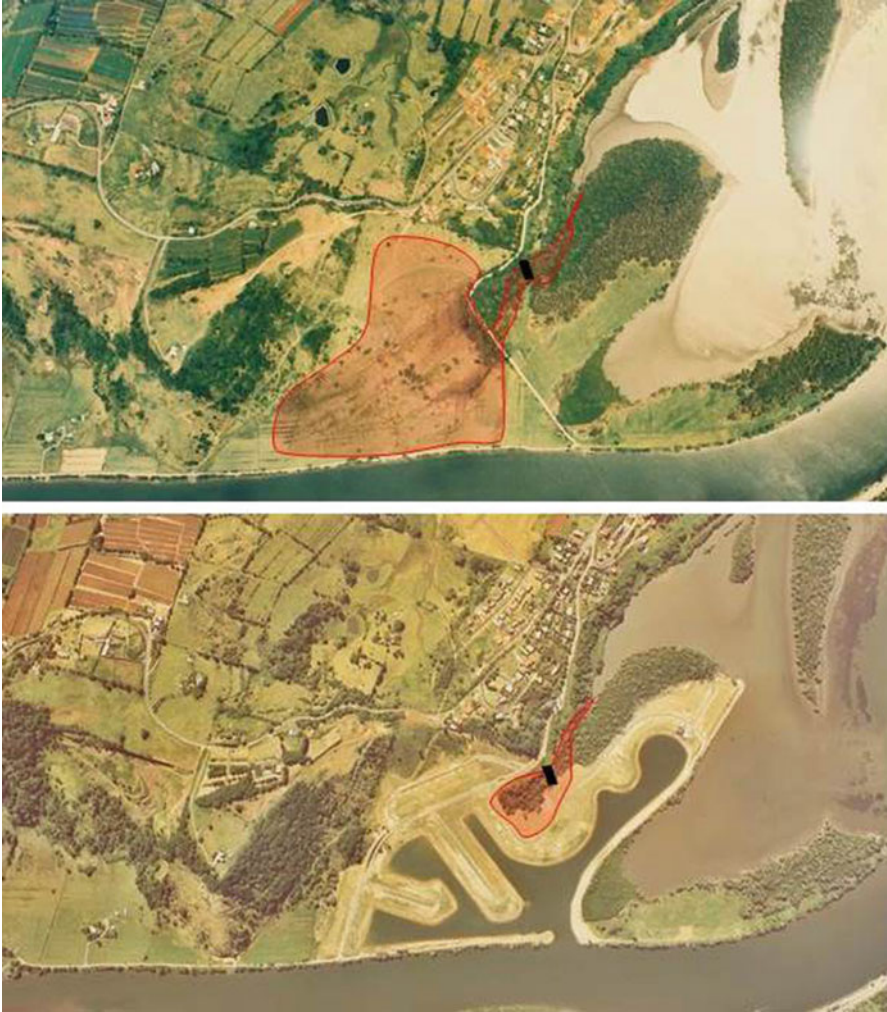
Fig. 33.4 Aerial photos from 1970s (top) and 1980s (bottom) showing the levee and catchment change that have contributed to the odour, poor water quality, weed incursion and mosquito hazard experienced by today’s residents
