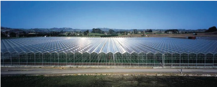
Fig. 4.9 Glass greenhouse in the peri-urban landscape of New Zealand
