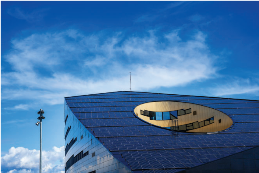
Figure 1. Powerhouse Brattørkaia - 'The World's Northernmost Energy-Positive Building'. Designed by Snøhetta, 2019. Photo: Erik Børseth. Reproduced with permission of Erik Børseth and Infinitiv AS. All rights reserved. The image is not covered by the CC-BY license and cannot be reused without permission.
