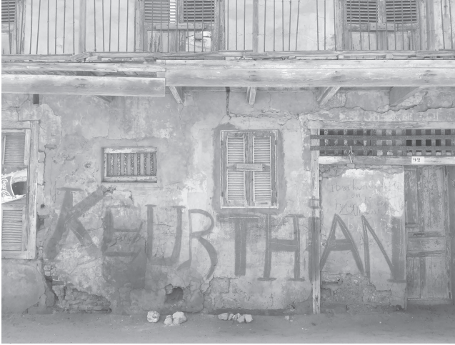
Figure 2.65 A house façade, Saint-Louis, Senegal.
