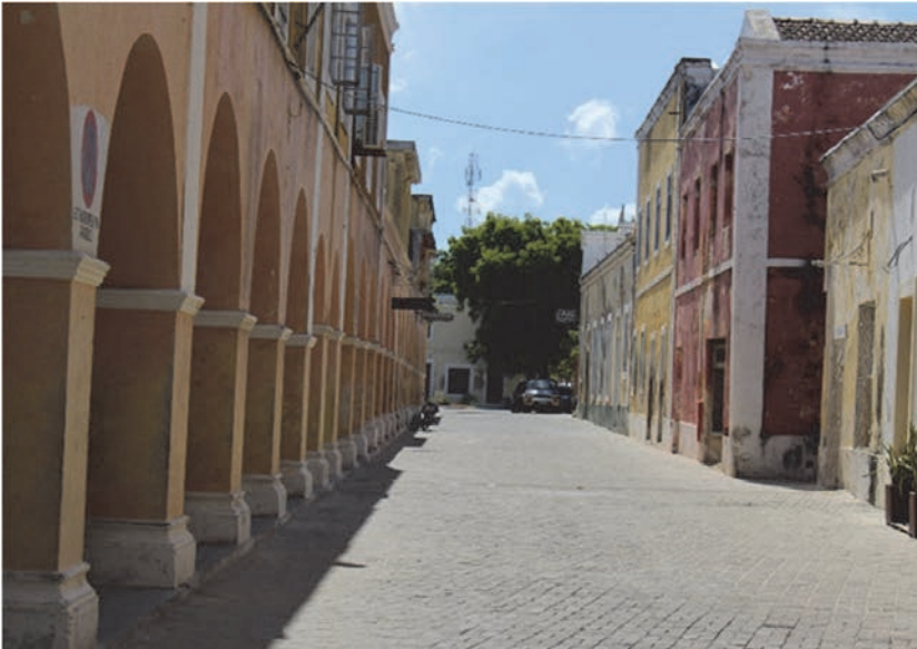
Figure 2: Street with arched colonnade in Ilha de Moçambique [Photo credit: Carla Bocchetti]
