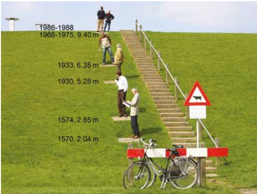
Figure 3.2 The Slachtedijk/Zeedijk at Oosterbierum. A number of stones mark past stages in the heightening of the dike.
