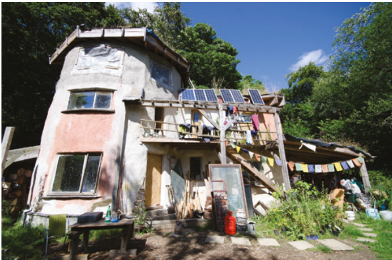
Figure 4.3 Almost complete straw bale and turf-roofed house at Green Hills (© Jenny Pickerill)
