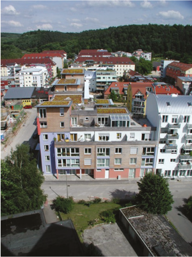
Figure 12.2 View over the rooftops of the French Quarter
