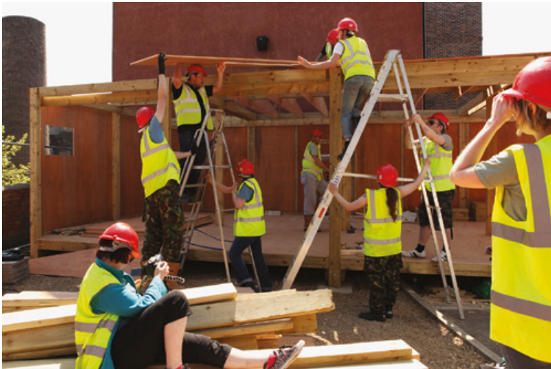
Figure 6.5 The site build (Photo credit: John Hipkin)
