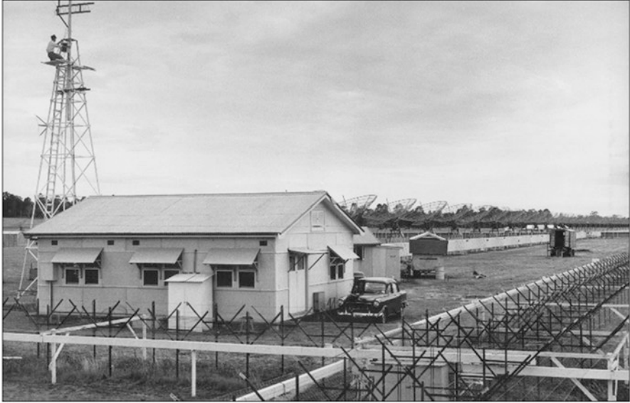
Fig. 2.60 Central area of the Mills Cross showing the receiver hut and the microwave antenna used for communicating with remote sites involved in interferometry (courtesy: CRAIA)
