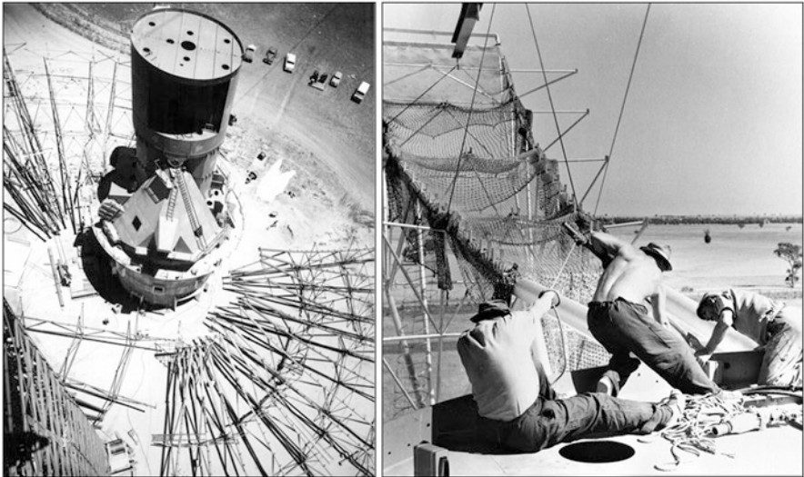
Fig. 5.3 The construction of the Parkes dish during 1959–1961 was carried out by the German steelmaker MAN. Most of the components of the telescope were cast at the MAN plant near Frankfurt and then shipped to Sydney (courtesy: CRAIA)
