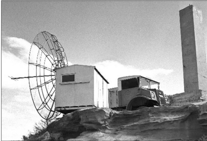
Fig. 2.18 The 3.9 m dish mounted in sea-interferometer mode on the back of an ex-Army truck (courtesy: CRAIA)
