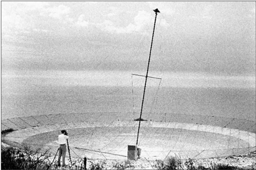
Fig. 2.24 The upgraded hole-in-the-ground antenna could survey consecutive strips of the sky by altering the position of the aerial mast. Here Gordon Stanley uses a theodolite to measure the mast's angle of tilt (courtesy: CRAIA)
