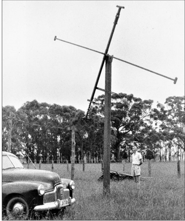
Fig. 2.49 Paul Wild with one of the simple position interferometer rhombic aerials. Because these aerials remained stationary, they did not require equatorial mounts (courtesy: CRAIA)
