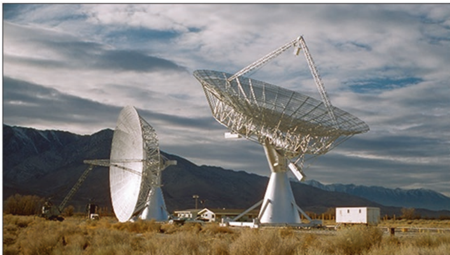
Fig. 1.22 In 1955 John Bolton and Gordon Stanley from Radiophysics were recruited by Caltech to establish a new radio astronomy group. They founded the Owens Valley Radio Observatory in northern California and designed an interferometer consisting of two 27 m dishes. The dishes were mounted on rail tracks so that the distance between the two could be varied (courtesy: Jim Roberts)
