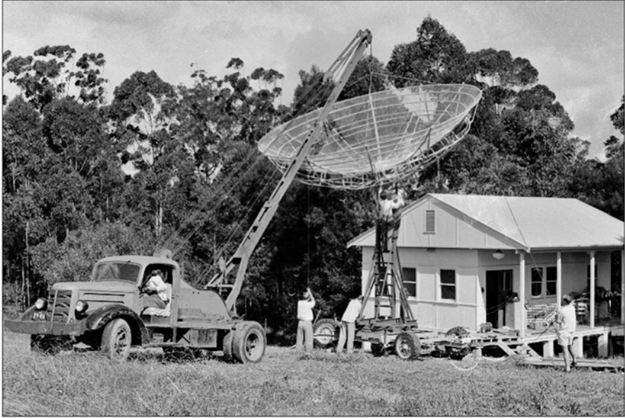
Fig. 2.68 Installation of the 6.4 m parabolic antenna and adjacent receiver hut at the Murraybank field station. This site in West Pennant Hills was located on an orchard belonging to John Murray's father, and so the name Murraybank (courtesy: CRAIA)
