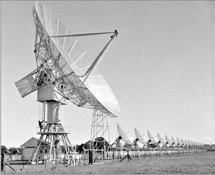
Fig. 2.66 View looking west showing the 18 m Kennedy Dish, installed at Fleurs in 1959, and some of the antennas in the E–W arm of the Chris Cross (courtesy: CRAIA)
