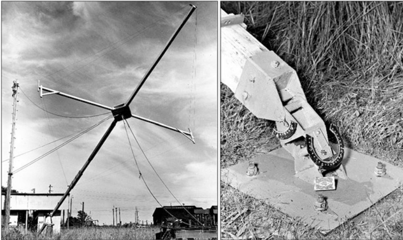
Fig. 2.45 (left) The rhombic antenna built by Paul Wild and Lindsay McCready at the Penrith field station. During 1949 this antenna operated with a swept-frequency spectrograph over a frequency range 70–130 MHz to study solar bursts. (right) The simple indicators used to point the antenna at the Sun at the start of each day’s observations (courtesy: CRAIA)
