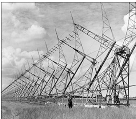
Fig. 1.39 Sir Martin Ryle was head of the Cambridge radio astronomy group and Director of the Mullard Radio Astronomy Observatory (after Hey, 1973: 64). The principal radio telescope by 1958 was an interferometer consisting of a parabolic cylinder reflector 475 m long and 20 m wide, and a smaller mobile reflector which could move along railway tracks (courtesy: CRAIA)
