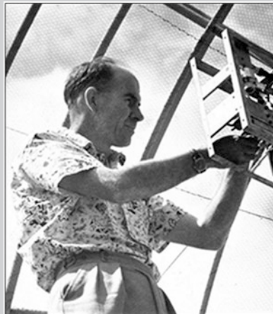
Fig. 4.32 Dick McGee working on the primary feed of the 6.4-m Murraybank antenna (courtesy: CRAIA)
