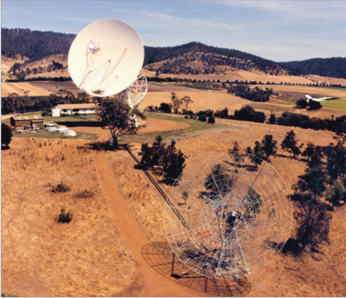
Fig. 5.22 The Physics Department at the University of Tasmania currently maintains two radio observatories, one at Mt Pleasant near Hobart (shown here), and the other at Ceduna on the Nullabor Plain (Fig. 5.21). At both stations, former US satellite-tracking 23 m dishes are the main antennas (courtesy: University of Tasmania and Martin George)
