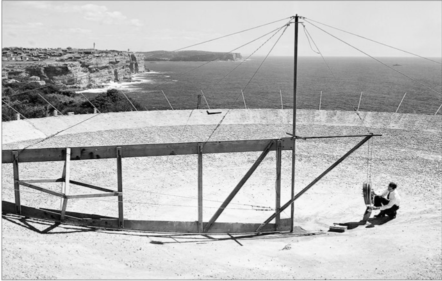
Fig. 2.23 Upgrading the hole-in-the-ground in February 1953 – a concrete surface was added and the diameter extended from 22 to 24.4 m. The rotating parabolic template was used to position formwork for the concrete and also to finish the surface (courtesy: CRAIA)
