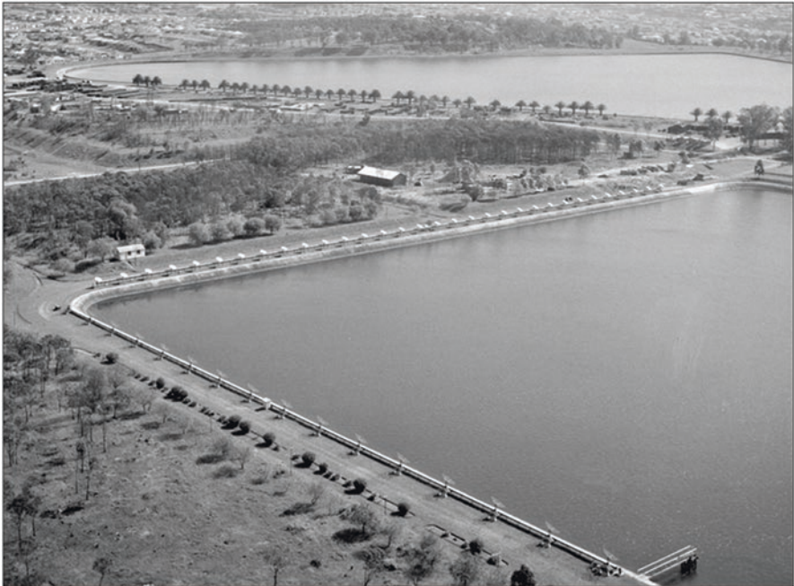
Fig. 2.33 Aerial view of the eastern reservoir at Potts Hill from the north, site of one of RP’s most productive field stations. Part of the larger, western water reservoir can be seen in the distance. The two 1420 MHz solar grating arrays are shown, with the original 32-element array in the background and the later 16-element array in the foreground (courtesy: CRAIA)
