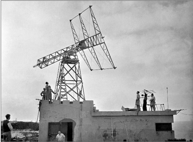
Fig. 2.17 The 9-Yagi array under construction early in 1949, with two of the Yagis leaning against the blockhouse. The array with its equatorial mount was used to carry out the first survey of the southern sky (courtesy: Stanley family)
