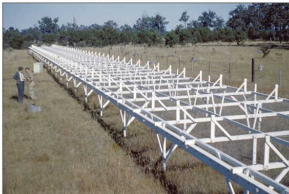
Fig. 4.26 The 50-dipole N–S array under construction at the Wallacia field station (courtesy: CRAIA)
