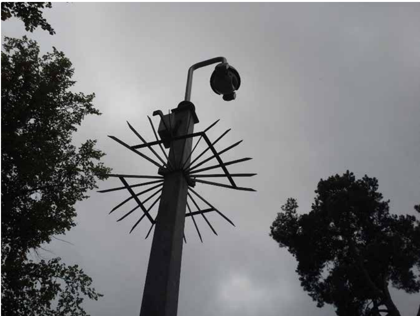
FIGURE 7.4 Outdoor security camera mounted on a pole and protected by pointed fencing, Winchester, England (photo by author).
