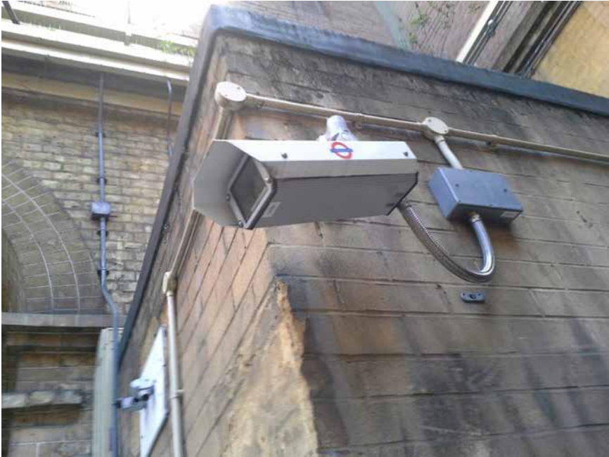
FIGURE 7.3 Tube platform security camera, London, England (photo by author).
